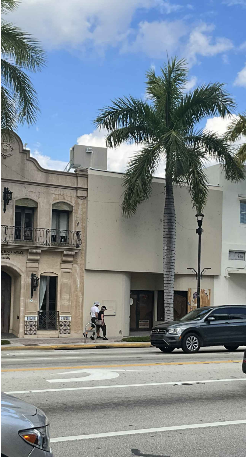
FRONT VIEW (SOUTH)
