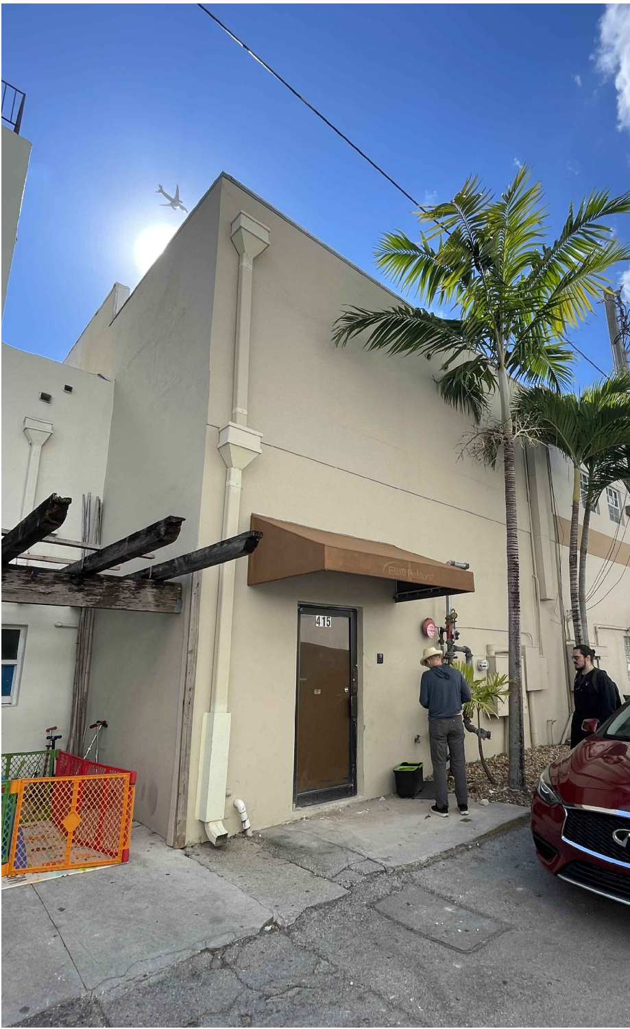
REAR VIEW (NORTH)
