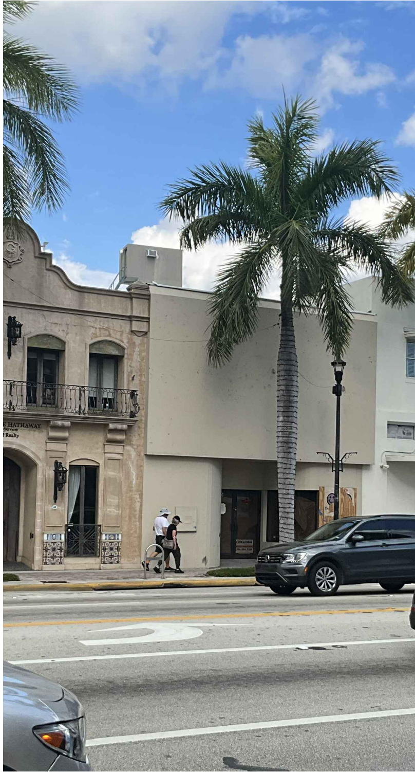
FRONT VIEW (SOUTH)
