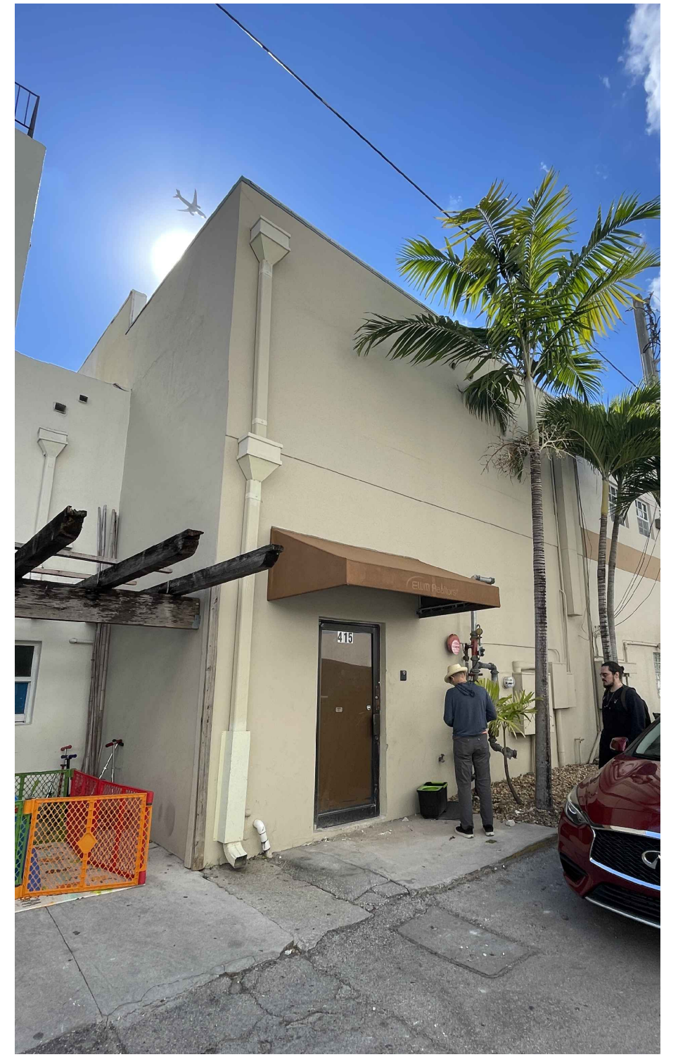
REAR VIEW (NORTH)
