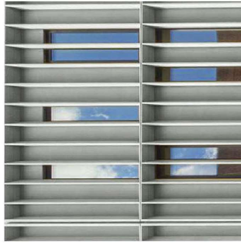
VERTICAL CONCRETE FINS at the lower volume of new addition
