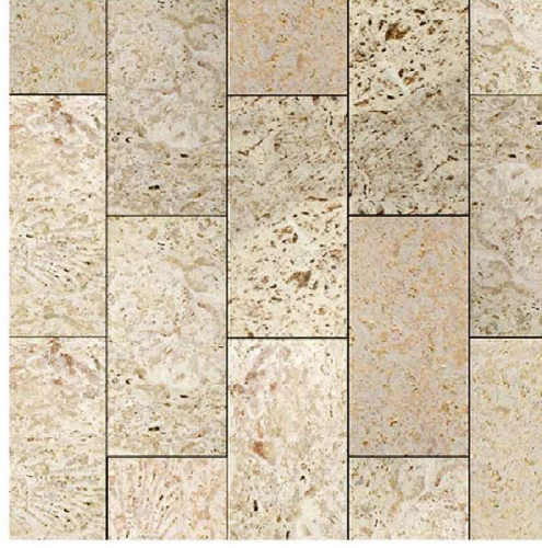
CORAL STONE WALL at the entry on Dickins Ave
