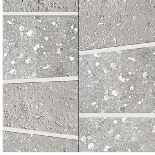
PRECAST PAVERS at the drop-off
