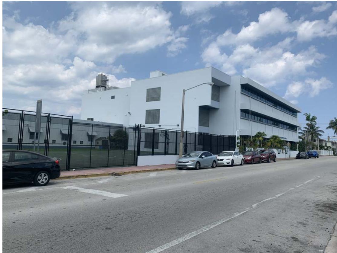
(1) VIEW FACING NORTHEAST ON 77th STREET
