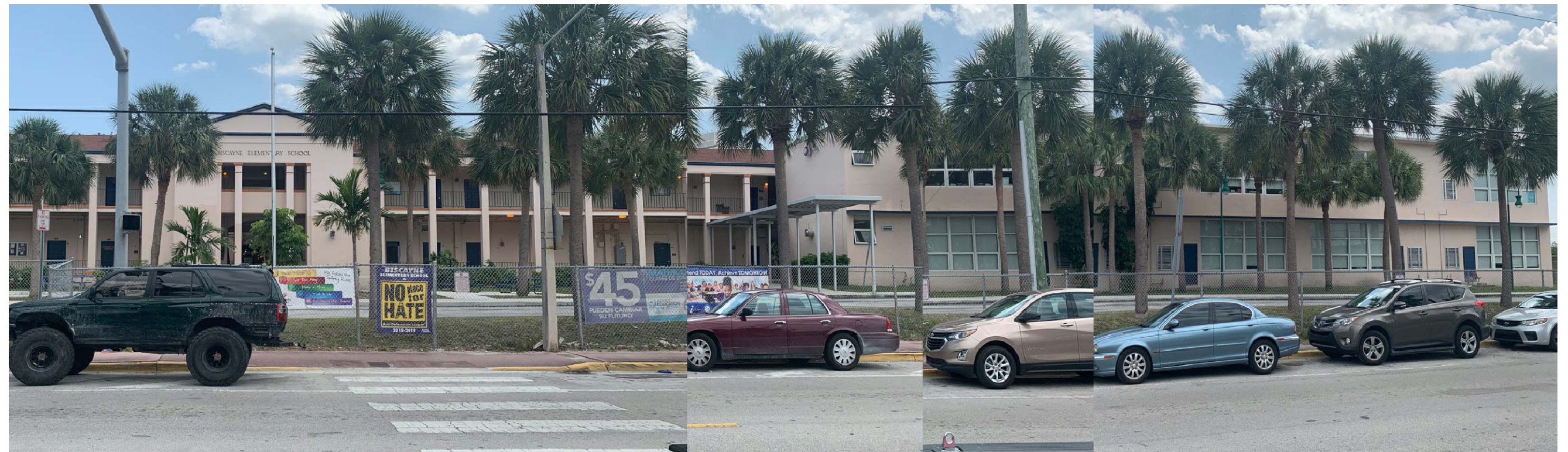
(2) VIEW FACING SOUTH ON 77th STREET
