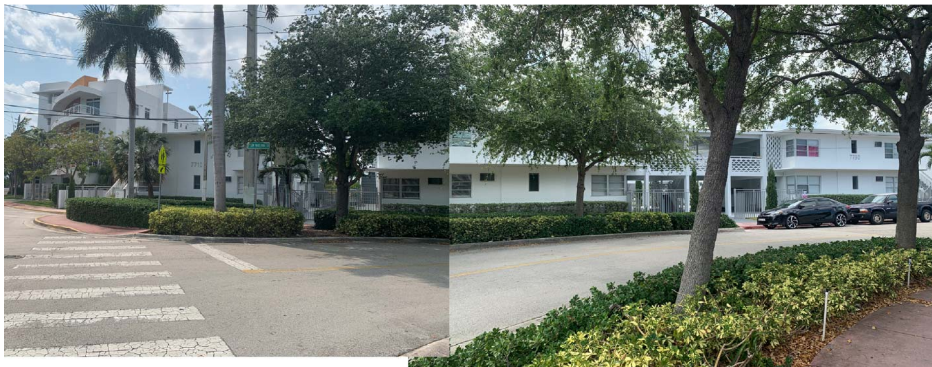
(1) VIEW FACING NORTHWEST ON 77th ST. & TATUM WATERWAY DRIVE
