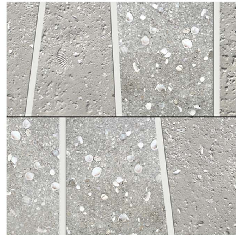
PRECAST PAVERS at the drop-off
