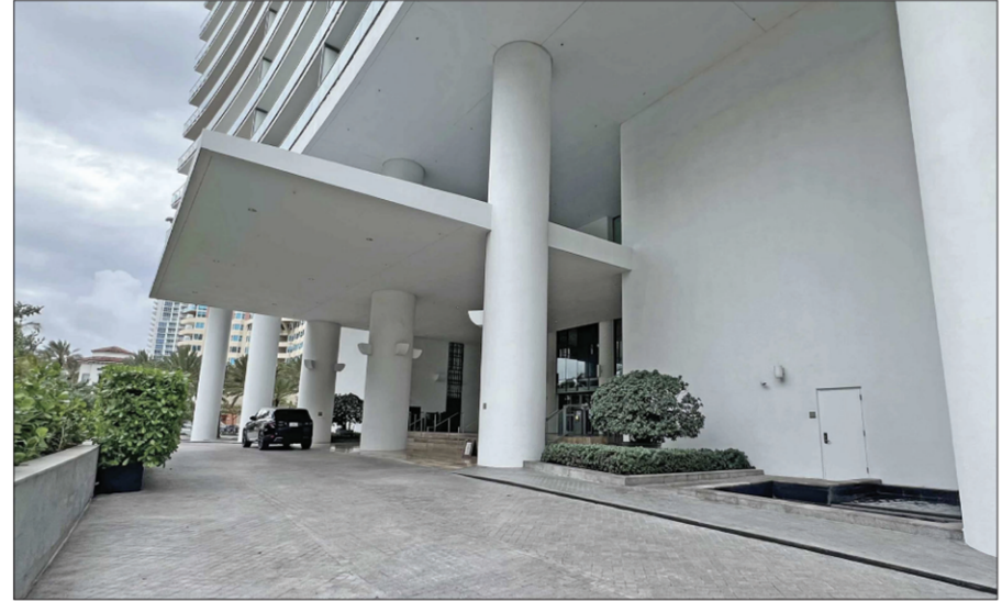
SITE VISIT 3/07/2025 2) VIEW EAST FROM ENTRY DRIVE TO PORTE COCHERE
