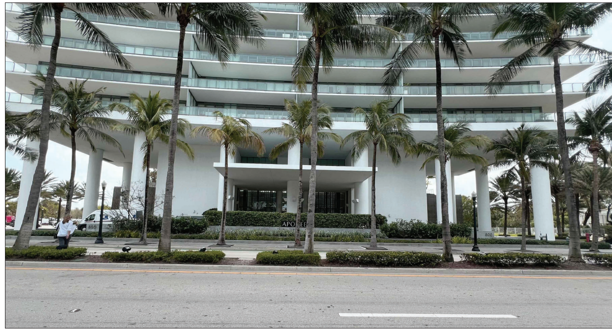
SITE VISIT 1/25/2024 3) VIEW OF NORTH ELEVATION
