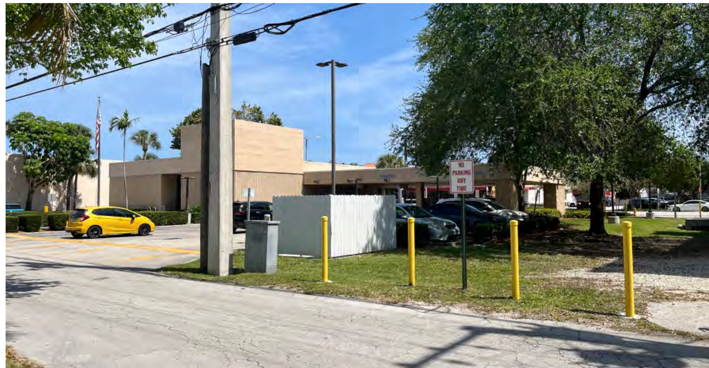
03 - VIEW OF EXISTING STRUCTURE FROM ALTON COURT - SOUTH
