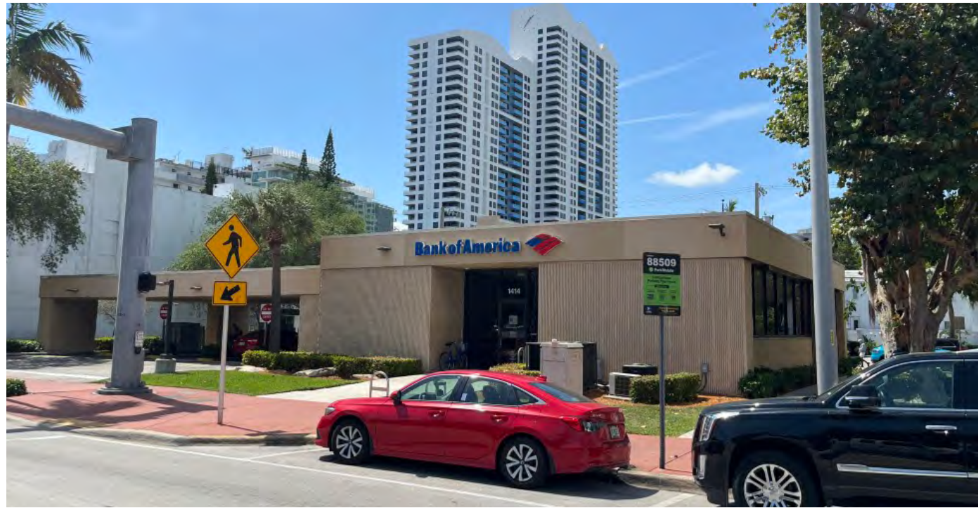
01 - VIEW OF EXISTING STRUCTURE FROM ALTON ROAD - NORTH
