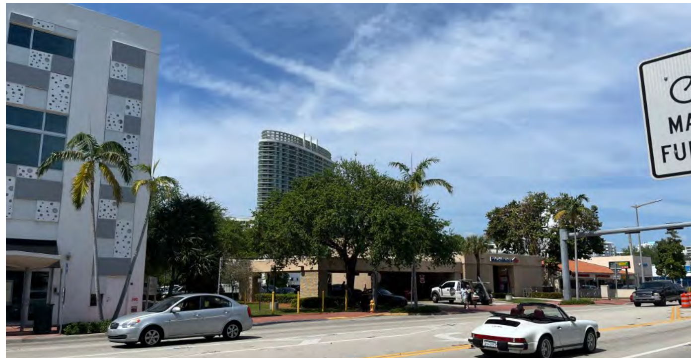
03 - VIEW OF EXISTING STRUCTURE FROM ALTON ROAD - SOUTH
