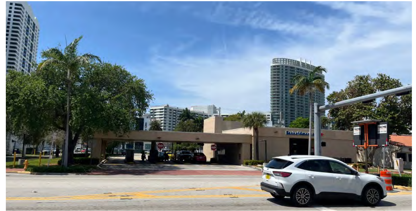
02 - VIEW OF EXISTING STRUCTURE FROM ALTON ROAD - EAST
