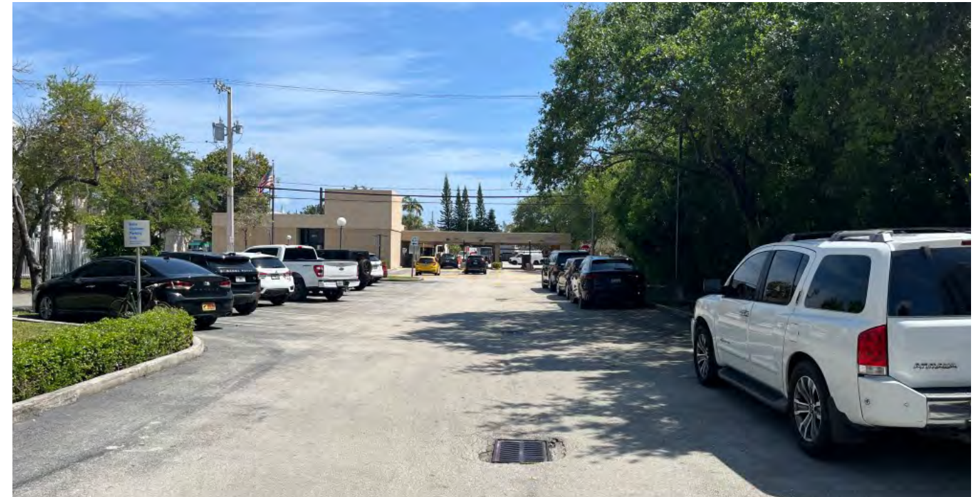
02 - VIEW OF EXISTING STRUCTURE FROM WEST AVE
