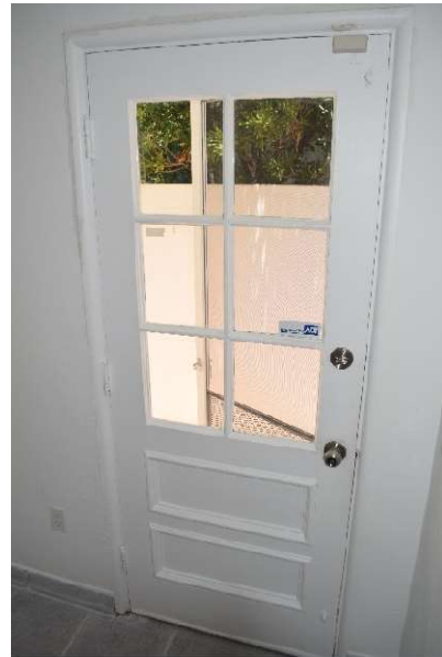
Figure 14. Exterior side door, May 2021.
