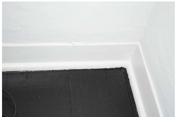
Figure 21. Wood base and flooring at Bedroom 1, May 2021.
