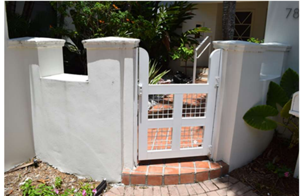
Figure 2 Wood gate adjacent driveway, May 2021.
