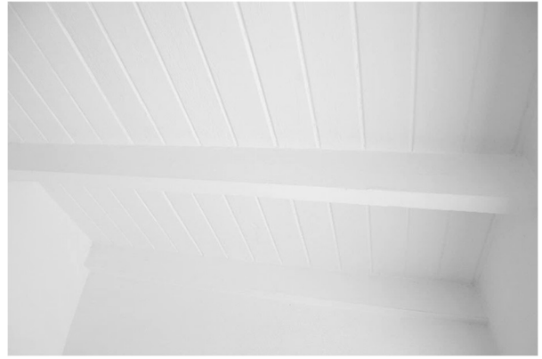
Figure 8. Tongue & groove ceiling at front porch, May 2021.
