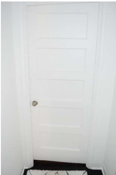
Figure 30. Interior door at Hall, May 2021.
