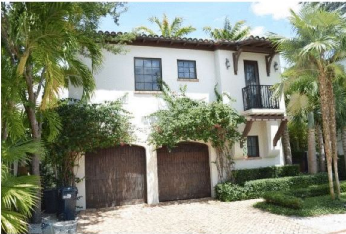
Figure 36. 7737 Atlantic Way (constructed 2012), May 2021.
