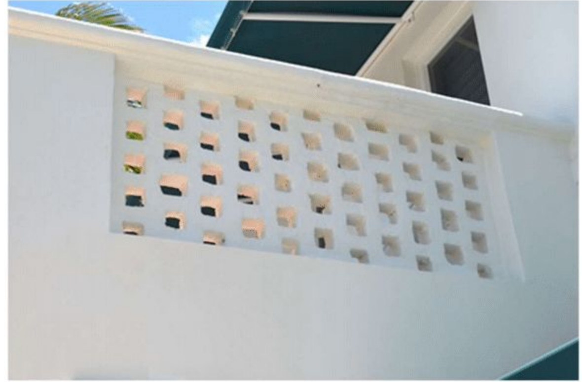
Figure 83. Detail of breezeblock at veranda, May 2021.
