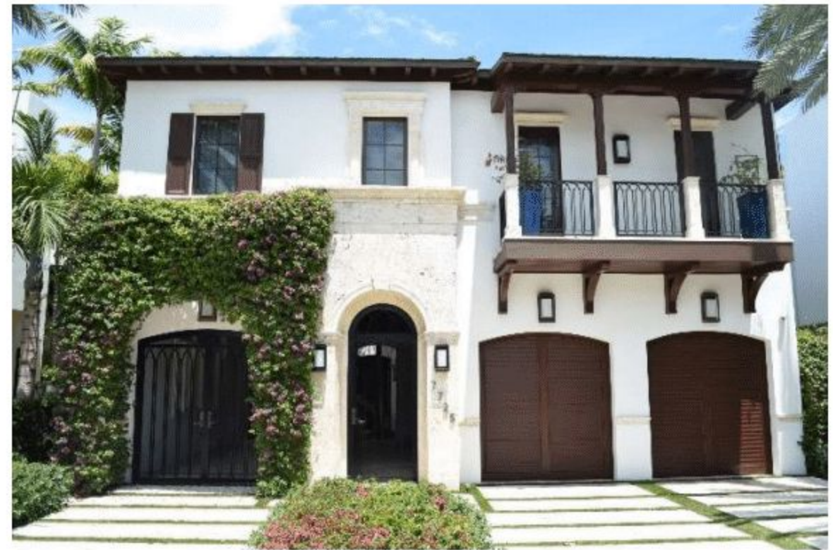
Figure 37. 7725 Atlantic Way (constructed 2012), May 2021.
