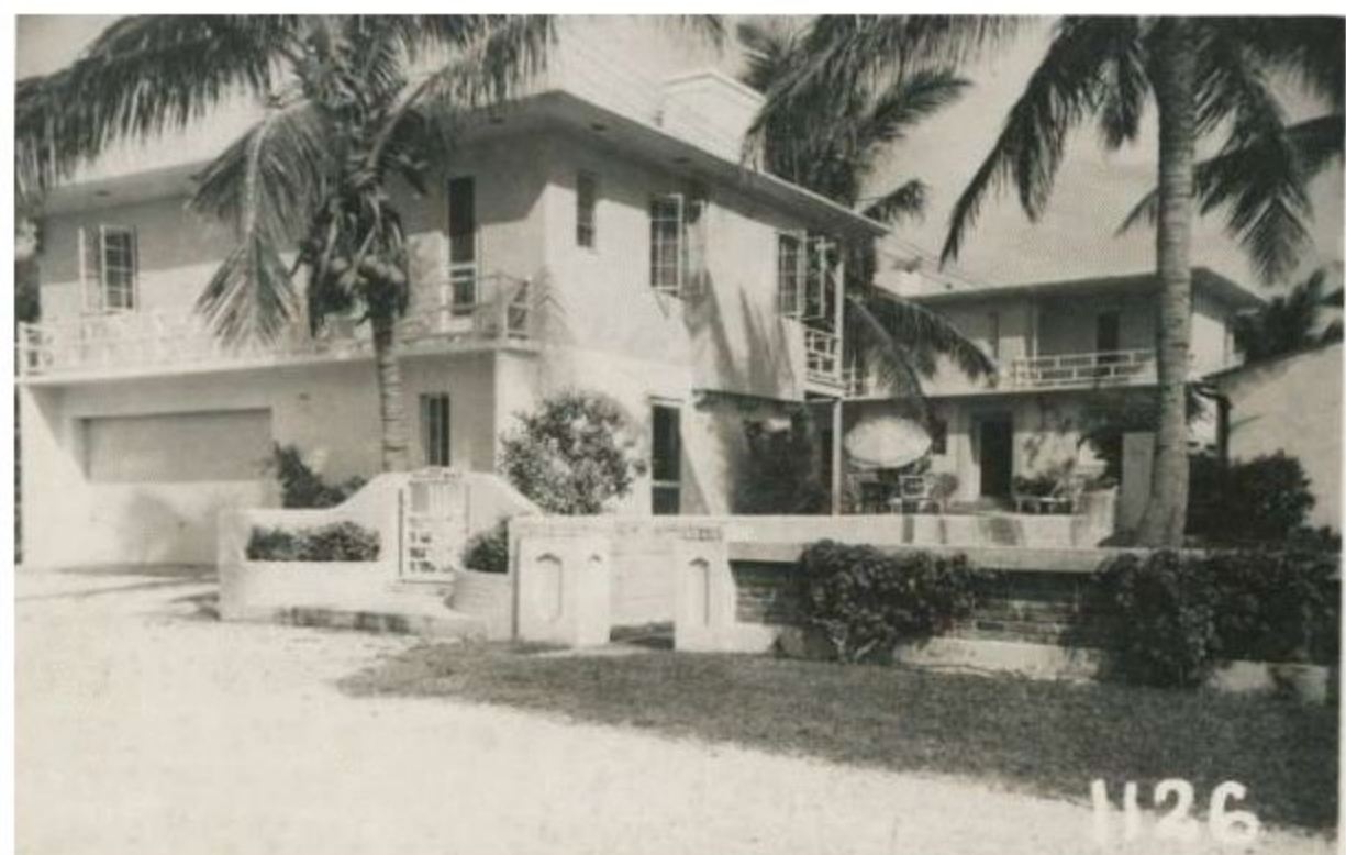
Figure 33. 7815 Atlantic Way (constructed 1936), October 1947. (Miami-Dade Public Library)
