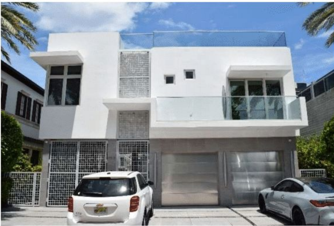
Figure 38. 7717 Atlantic Way (constructed 2017), May 2021.
