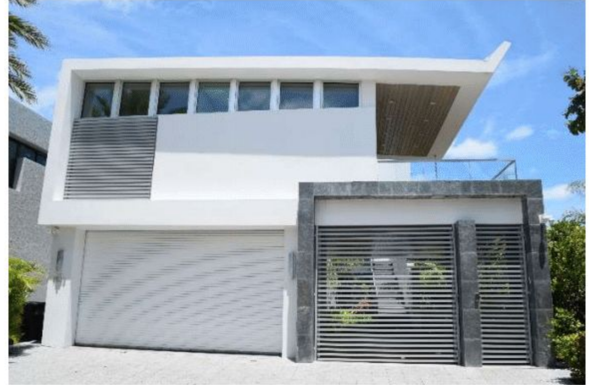
Figure 29. 7833 Atlantic Way (constructed 2019), May 2021.
