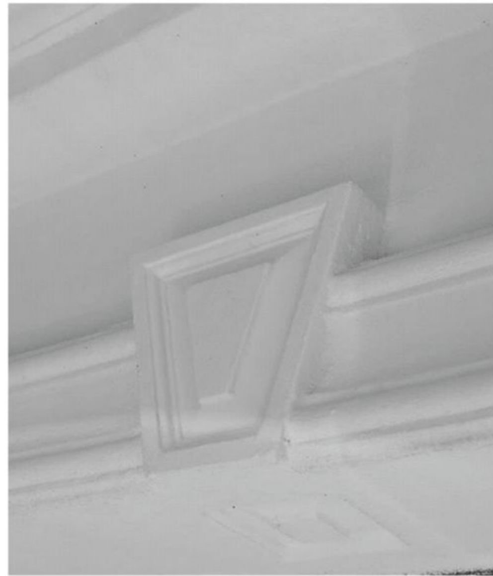
Figure 81. Detail of keystone at garage door, May 2021.
