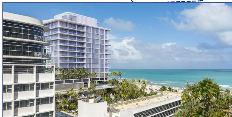
7. Ground Up Addition
