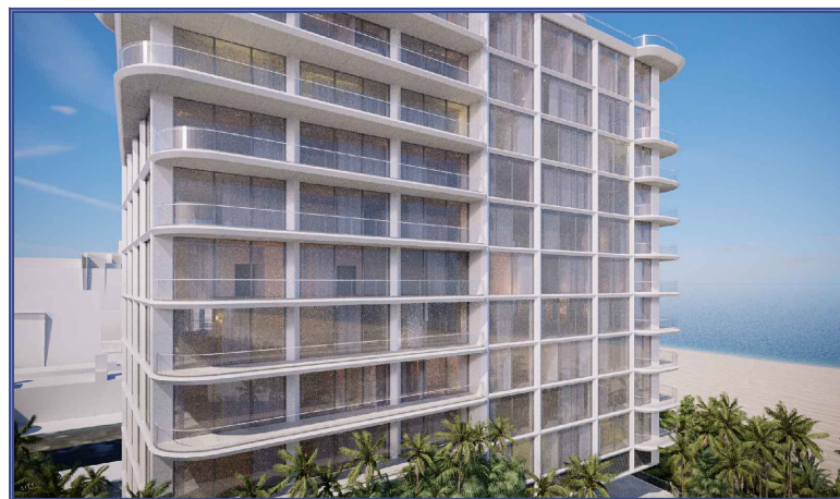
9. New Building balconies
