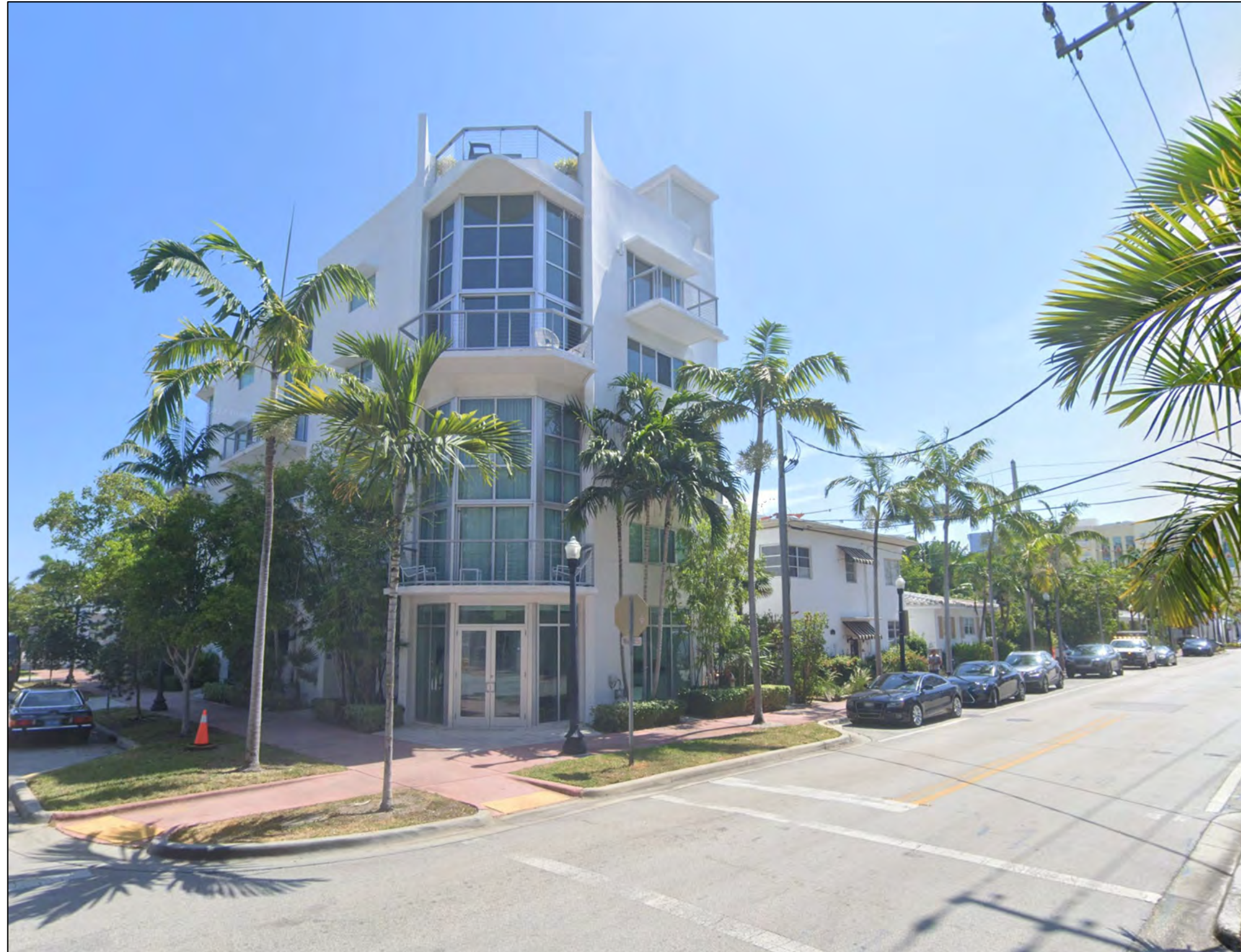
8. STREET VIEW -NORTH SIDE FACING NE
