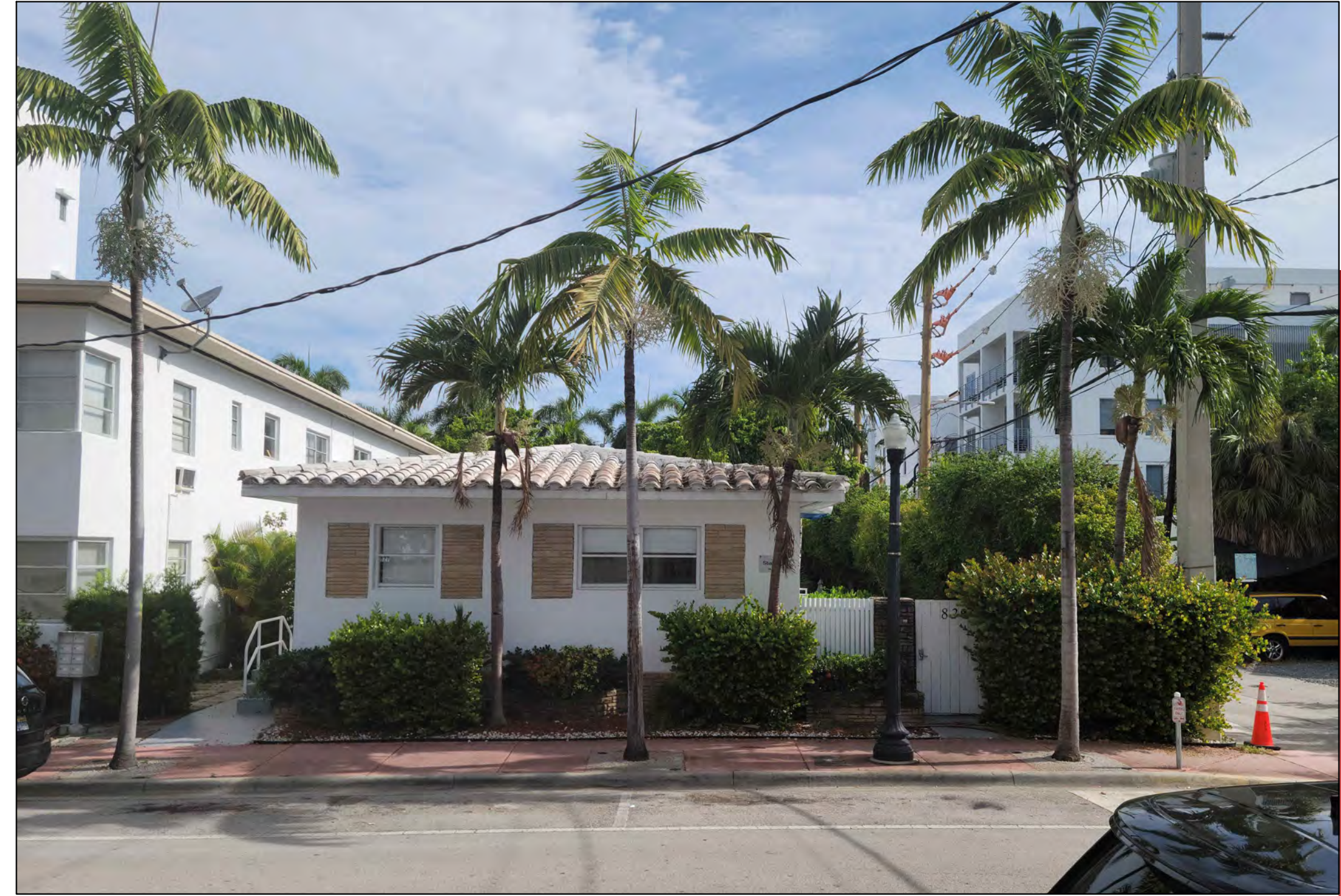
15. STREET FACADE VIEW @ 4TH STREET
