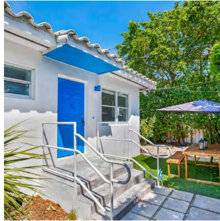
STAIR STOOP AND HANDRAILS
