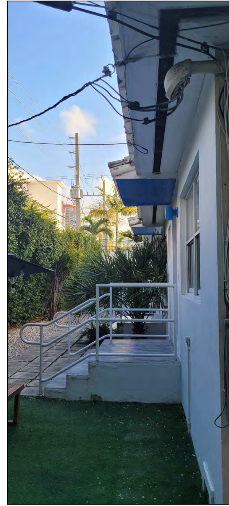
STAIRS STOOPS AND RAILINGS TO BE DEMOLISHED
