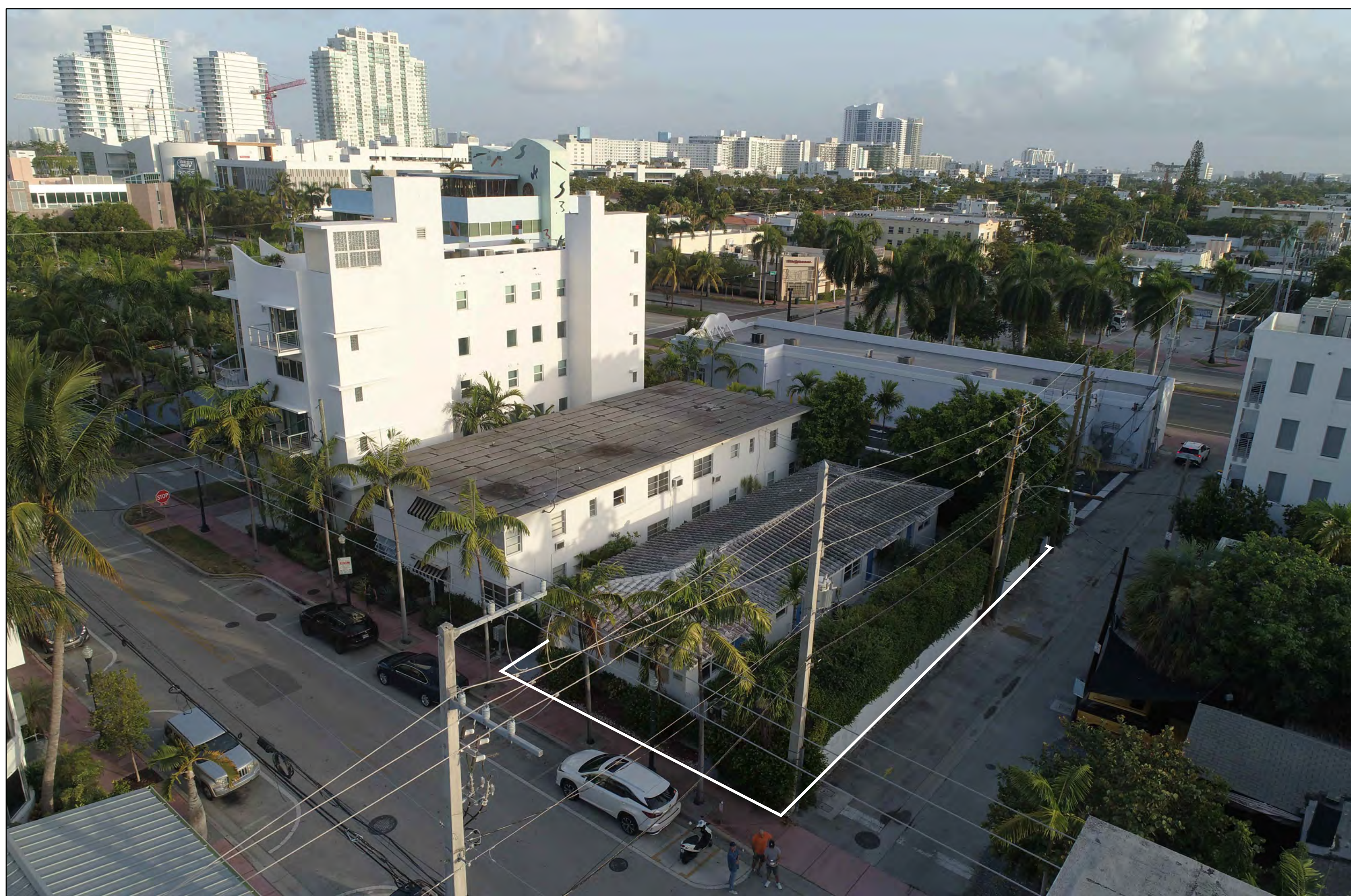
6. AERIAL VIEW OF 829 4TH STREET FACING NW
