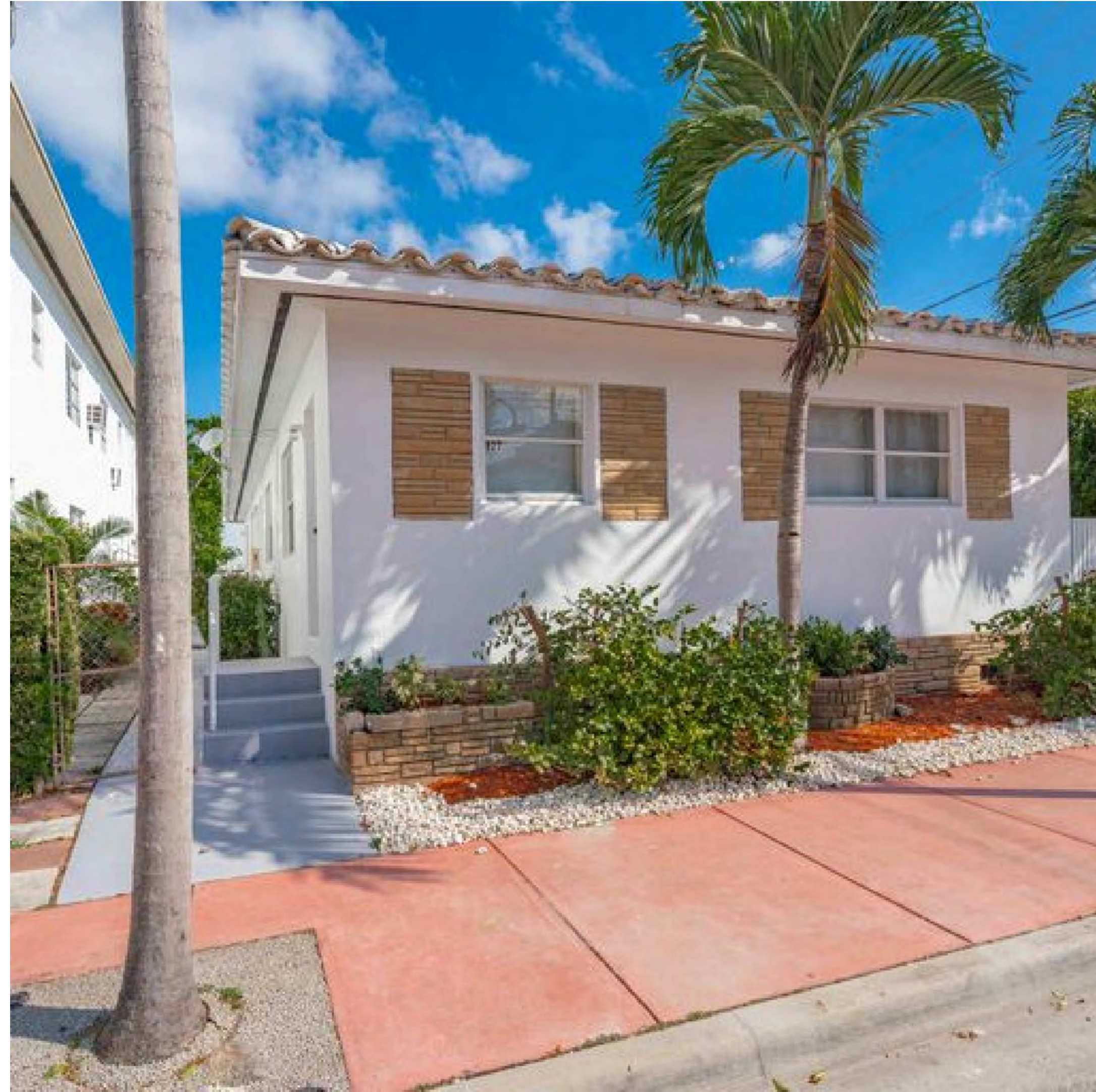
14. STREET FACADE VIEW @ 4TH STREET
