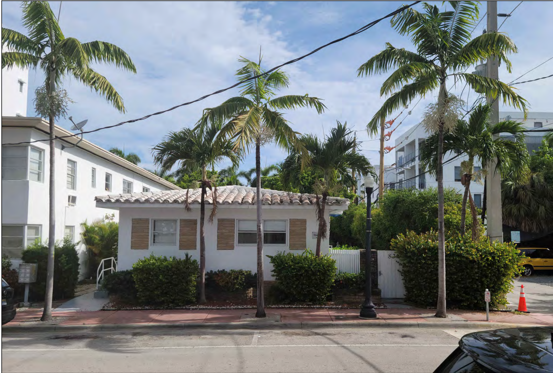
15. STREET FACADE VIEW @ 4TH STREET
