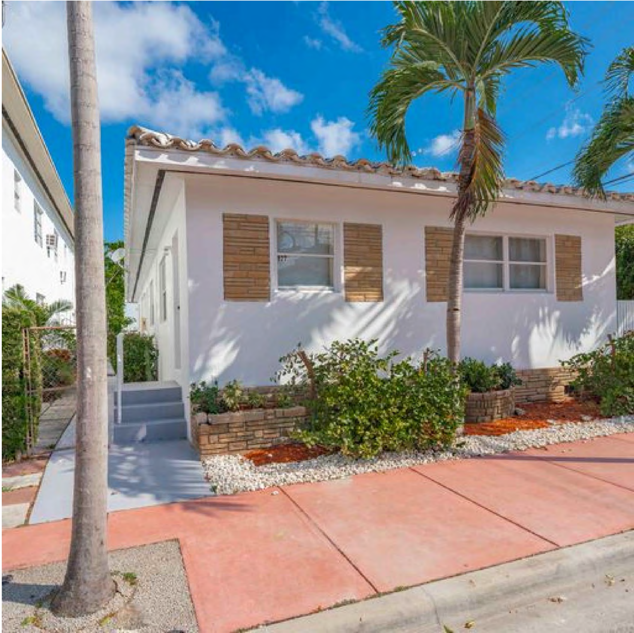
14. STREET FACADE VIEW @ 4TH STREET
