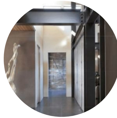
EXPOSED STEEL COLUMNS AND BEAMS
