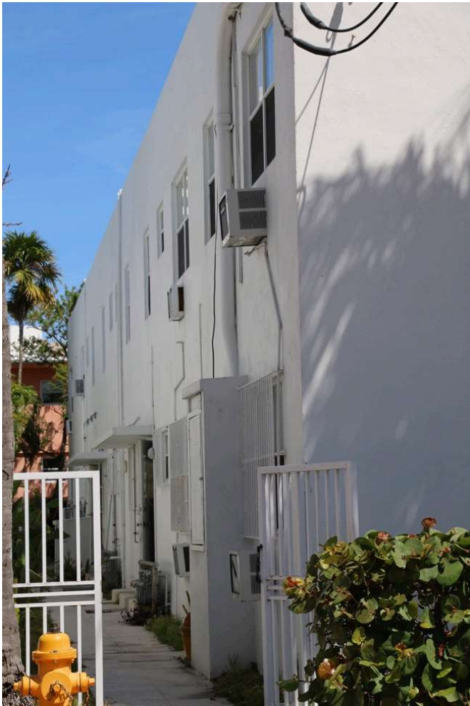
TOP LEFT PHOTO: 2018 PHOTOGRAPH OF NORTHERN ELEVATION (7)
