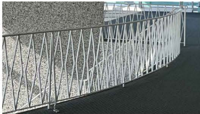
INTERIOR BALCONY EXISTING PHOTO
