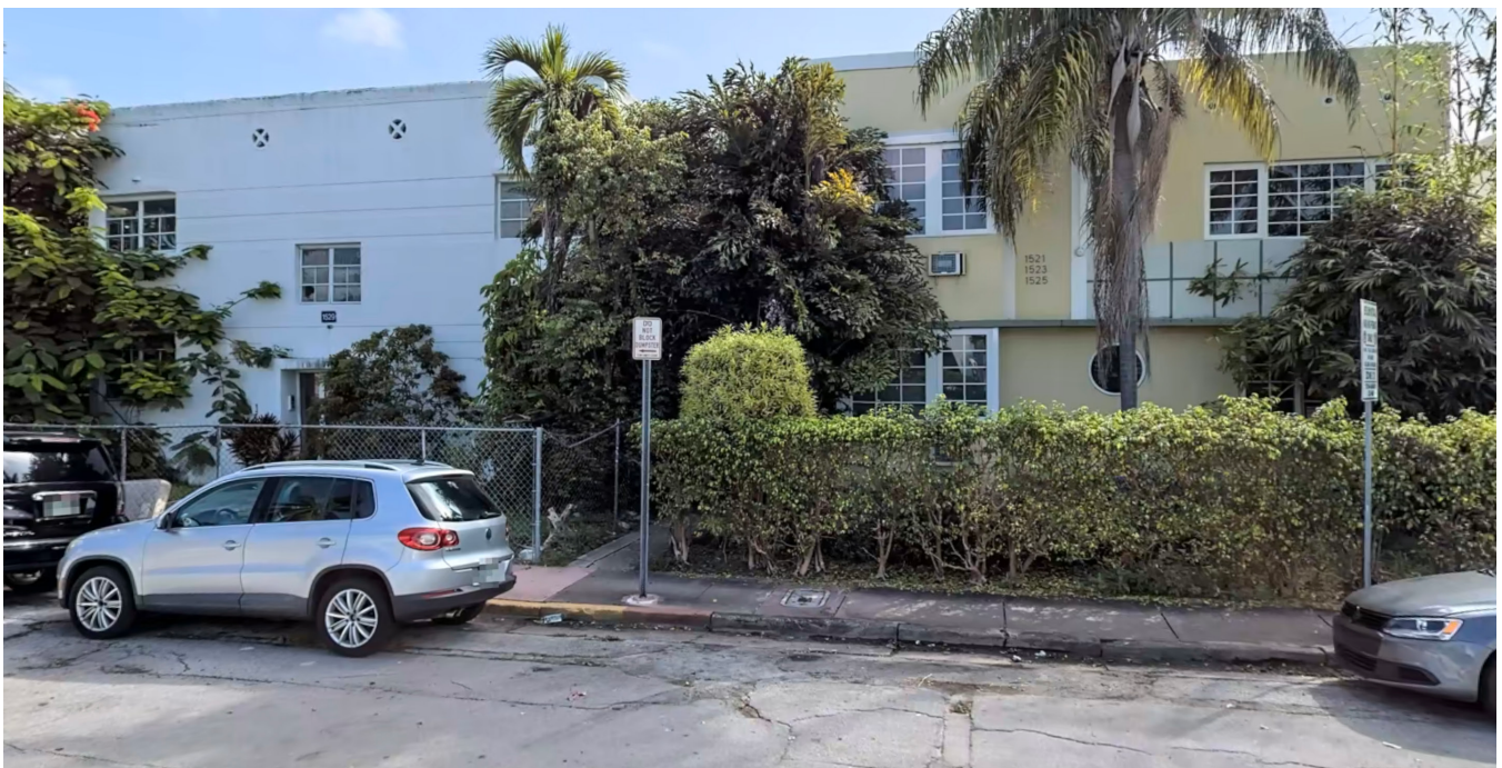
Surrounding Context to the South
