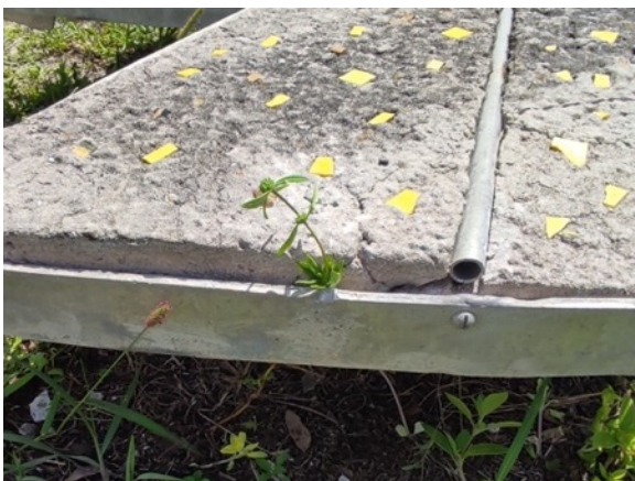
Detail of hollow, superficial aluminum decorative tube on 'ground' panel.
