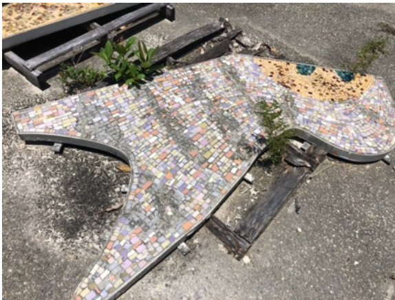
Overall of panel #20 before relocation.
