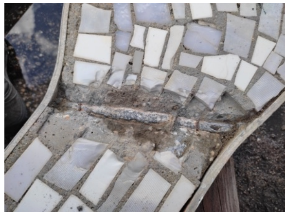
Detail of excavated aluminum tube showing internal corroded ferrous bar, and corroded wires (supposedly attached to mesh) at panel #4.
