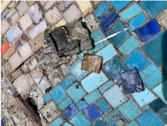
Detail of panel #1, showing dislodged tiles with bio growth visible on both the backs of the tiles as well as on the bedding mortar over which they sat.
