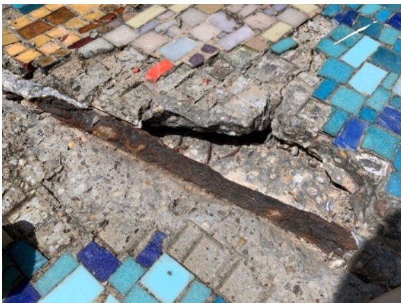
Detail of exposed aluminum tube, corroded ferrous bar, corroded wire mesh, and large cavity at panel #1.
