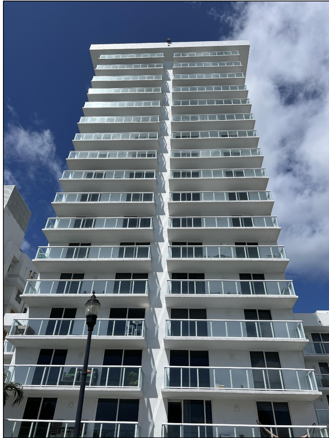
2457 COLLINS AVE. REAR OF BUILDING EAST FACADE 03/28/2023
