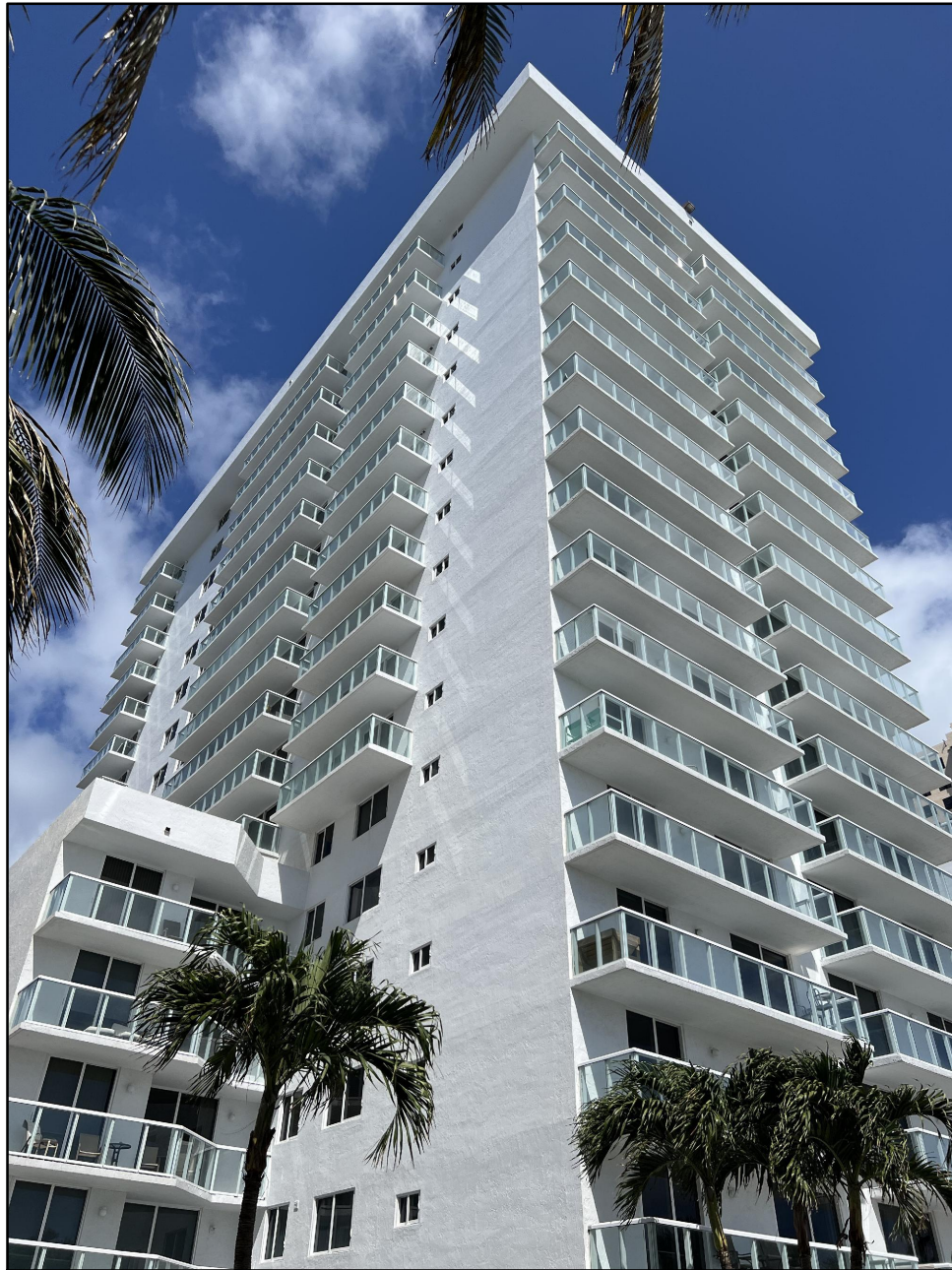
2457 COLLINS AVE. REAR OF BUILDING EAST AND SOUTH FACADE 03/28/2023
