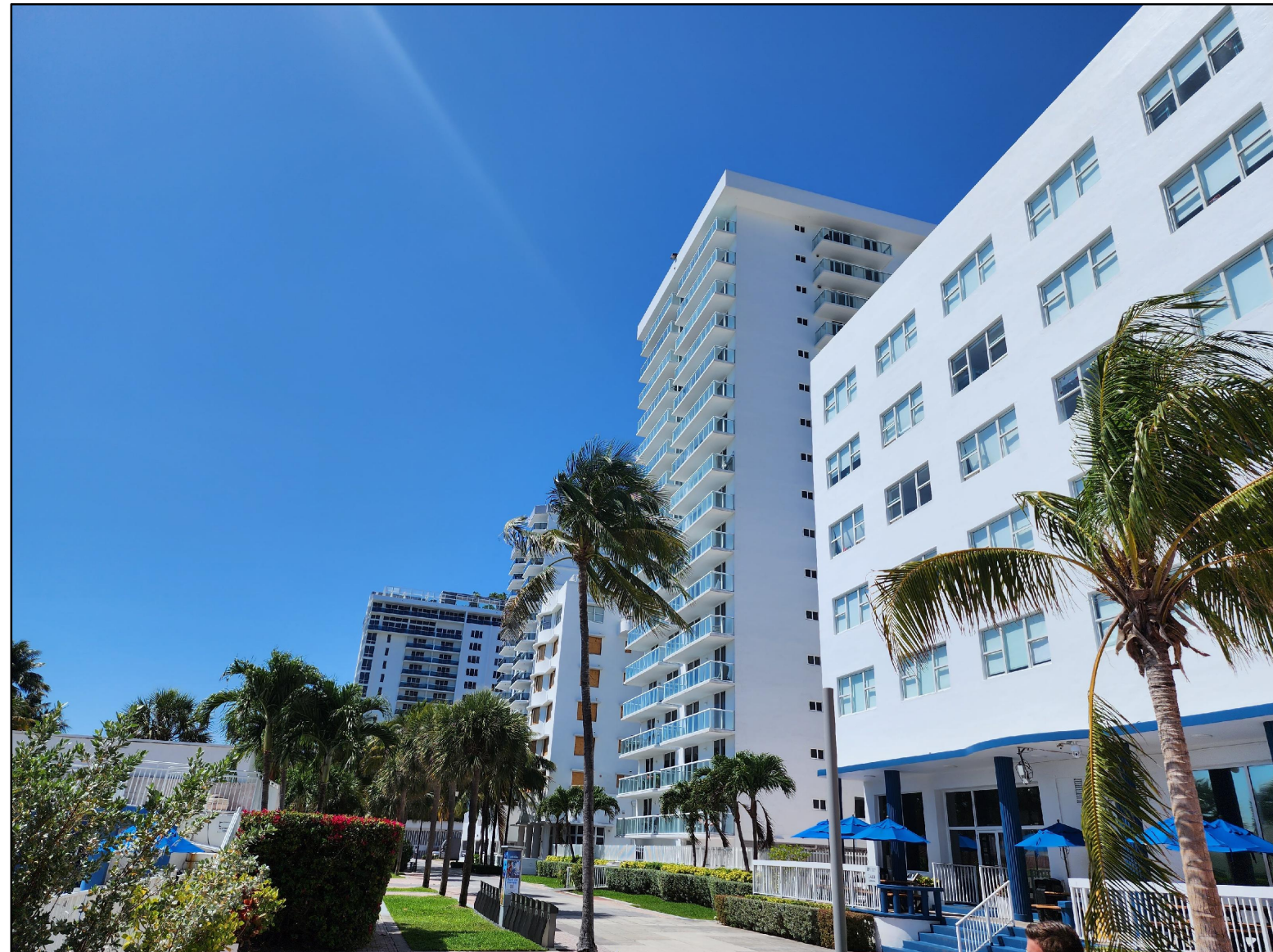
2457 COLLINS AVE. REAR OF BUILDING EAST FACADE 03/28/2023
