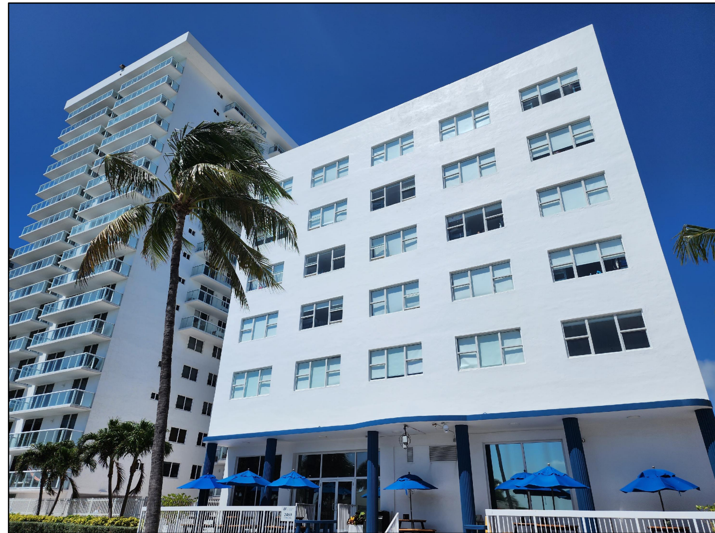
2457 COLLINS AVE. REAR OF BUILDING EAST FACADE 03/28/2023
