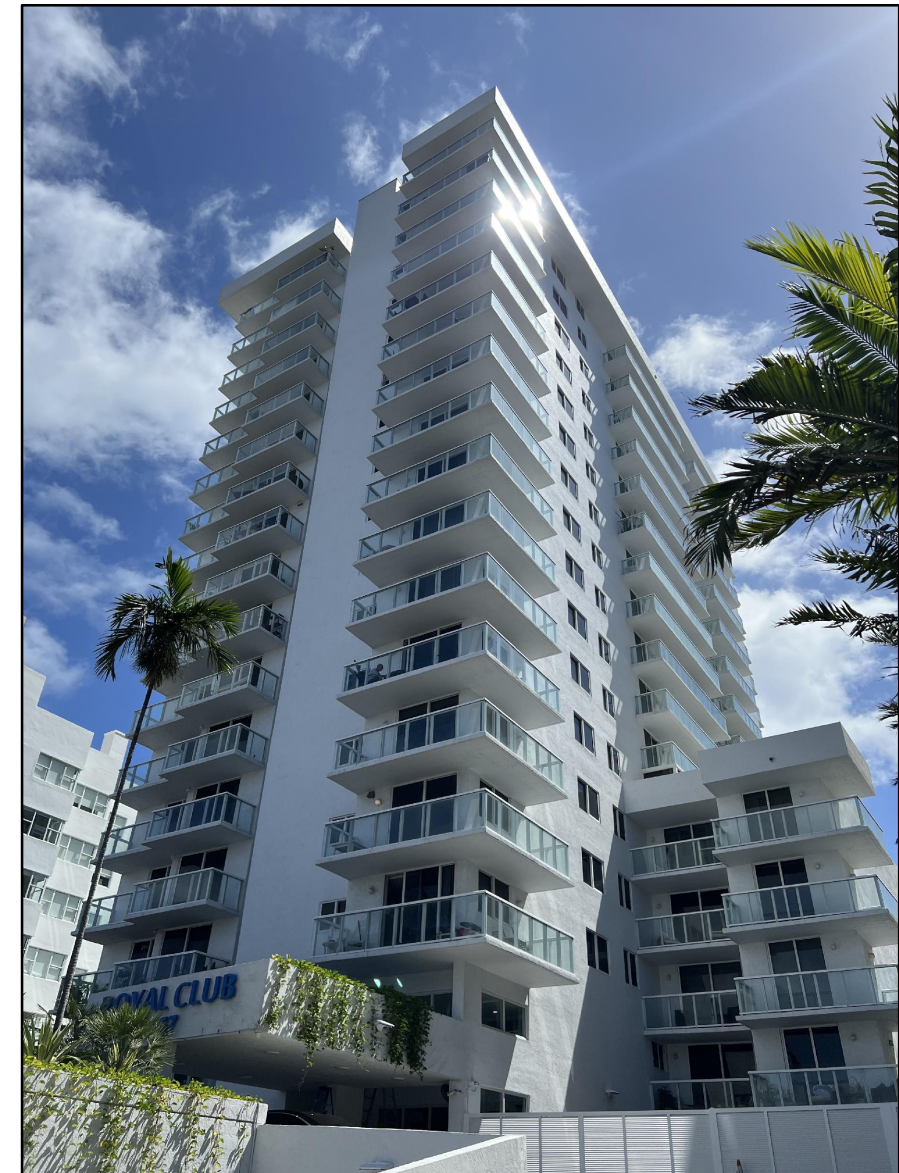
2457 COLLINS AVE. FRONT OF BUILDING WEST AND SOUTH FACADE 03/28/2023
