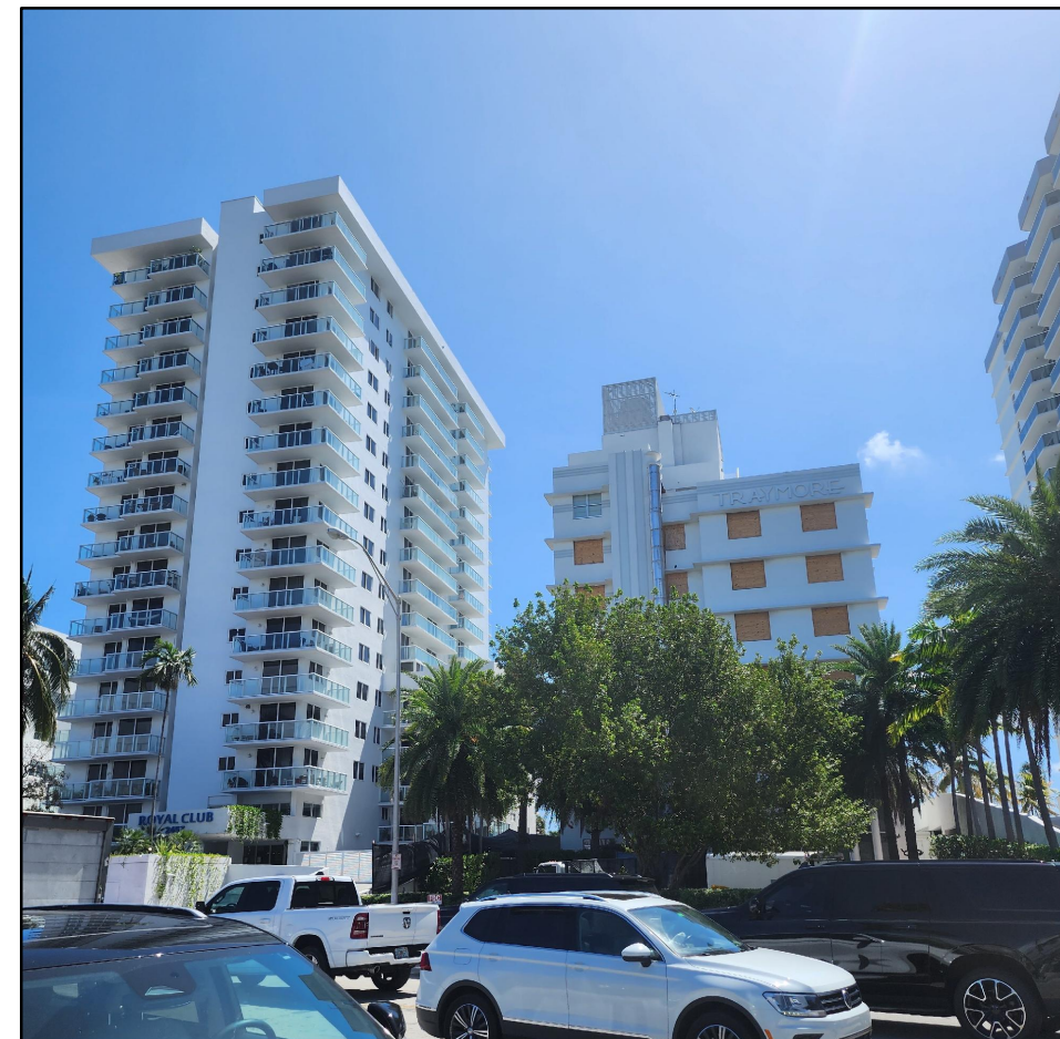
2457 COLLINS AVE. FRONT OF BUILDING WEST AND SOUTH FACADE 03/28/2023
