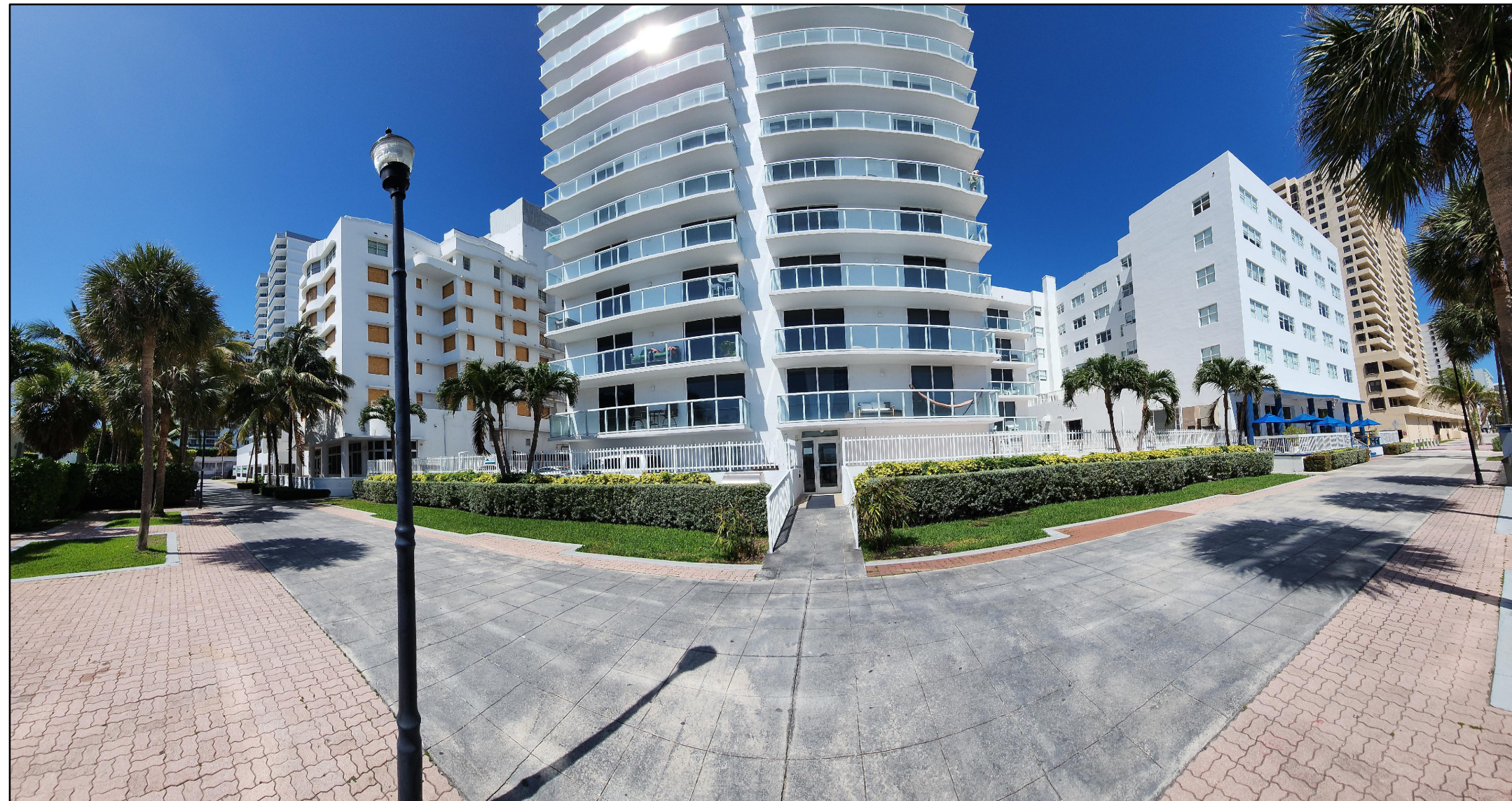
2457 COLLINS AVE. REAR OF BUILDING EAST FACADE 03/28/2023
