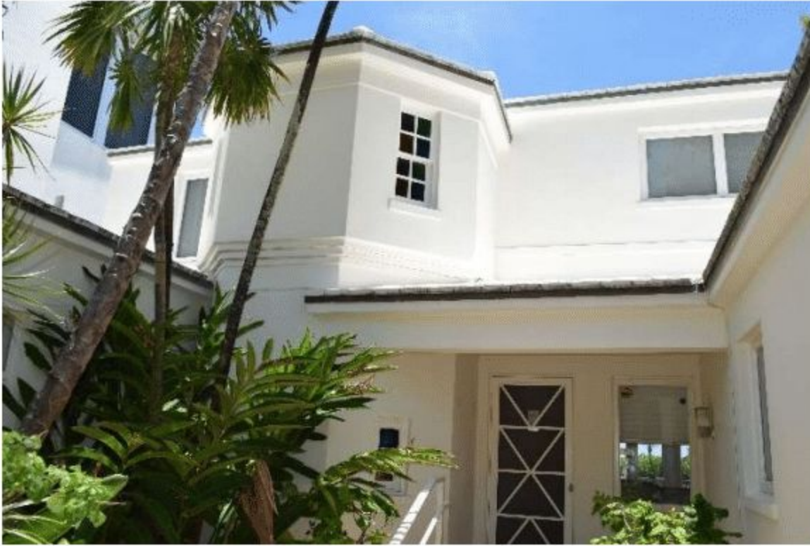
Figure 74. View of west elevation, May 2021.
