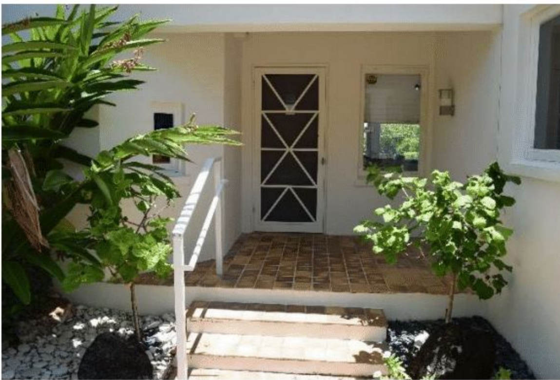
Figure 76. Detail of front entrance, May 2021.
