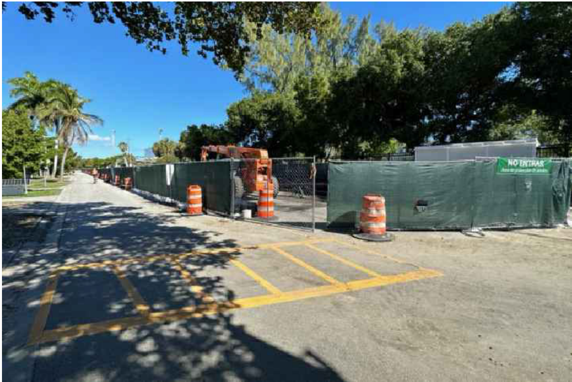
5. FPL WORK ON MICHIGAN AVENUE
