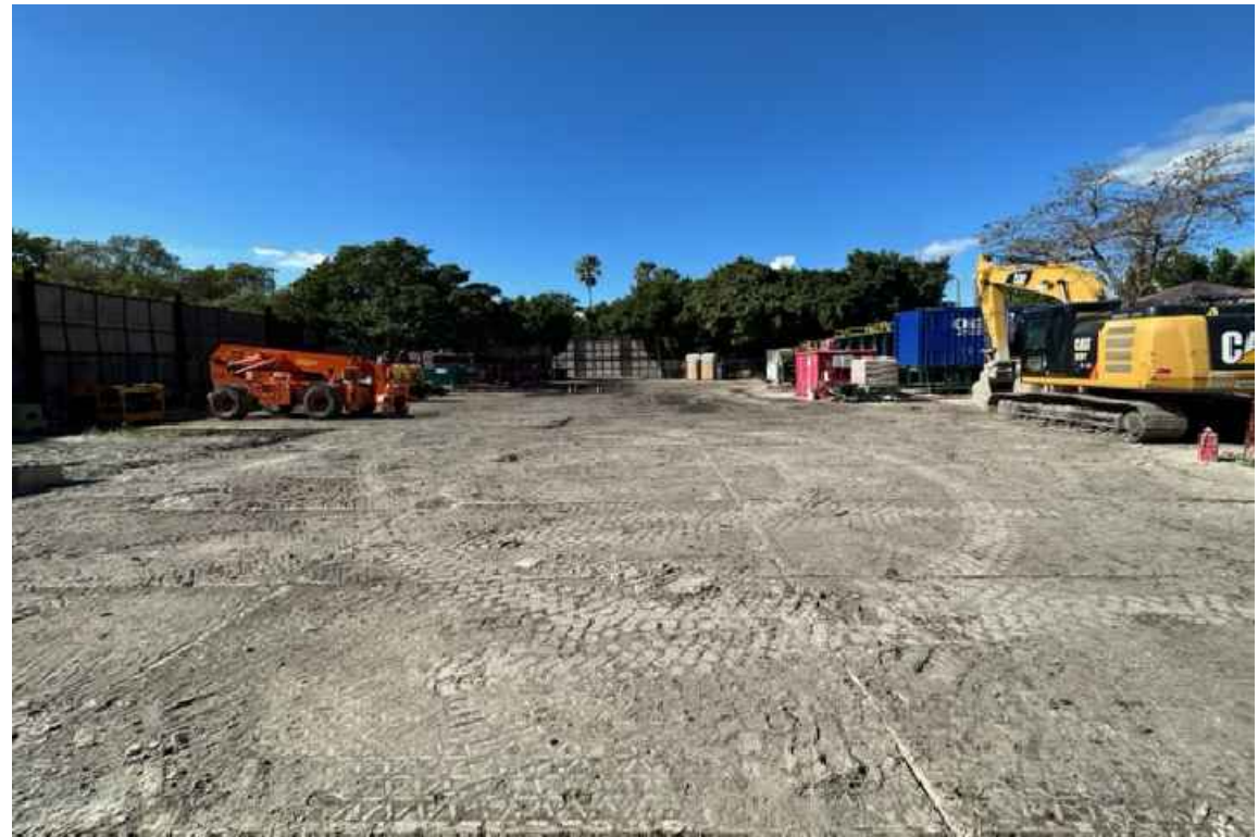
15. INSIDE FPL STAGING AREA FACING MICHIGAN AVENUE
