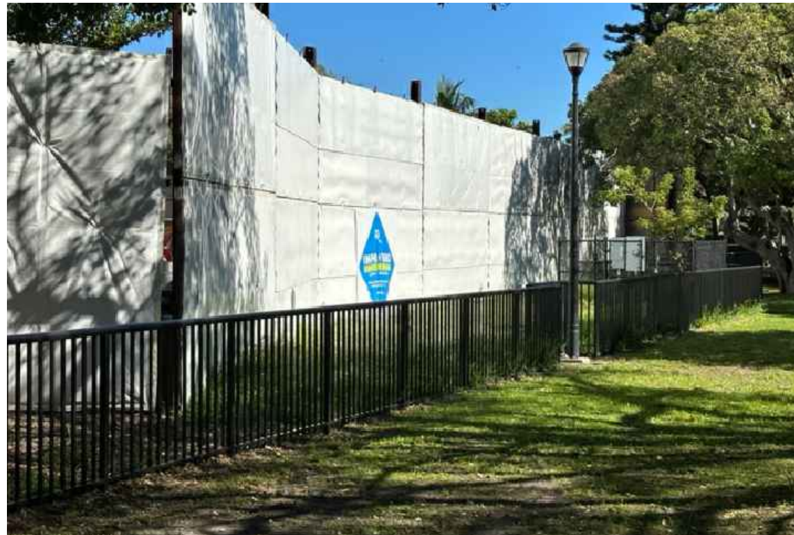
11. FENCE BETWEEN PLAYGROUND AND FPL STAGING AREA, ELECTRICAL PANEL AND METER TOWARDS THE BACK
