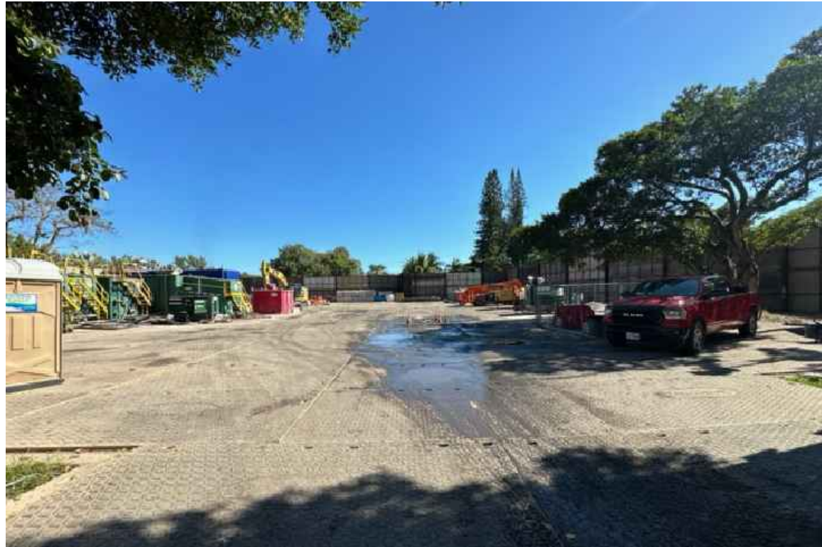
13. INSIDE FPL STAGING AREA
