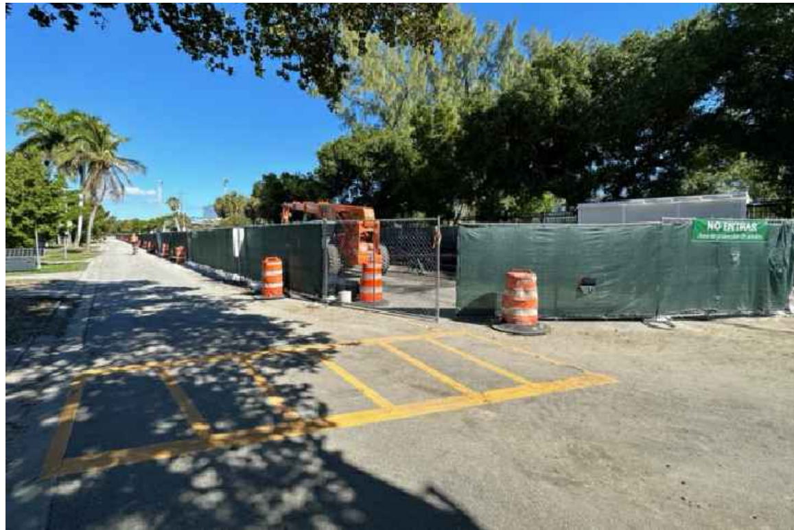
5. FPL WORK ON MICHIGAN AVENUE
