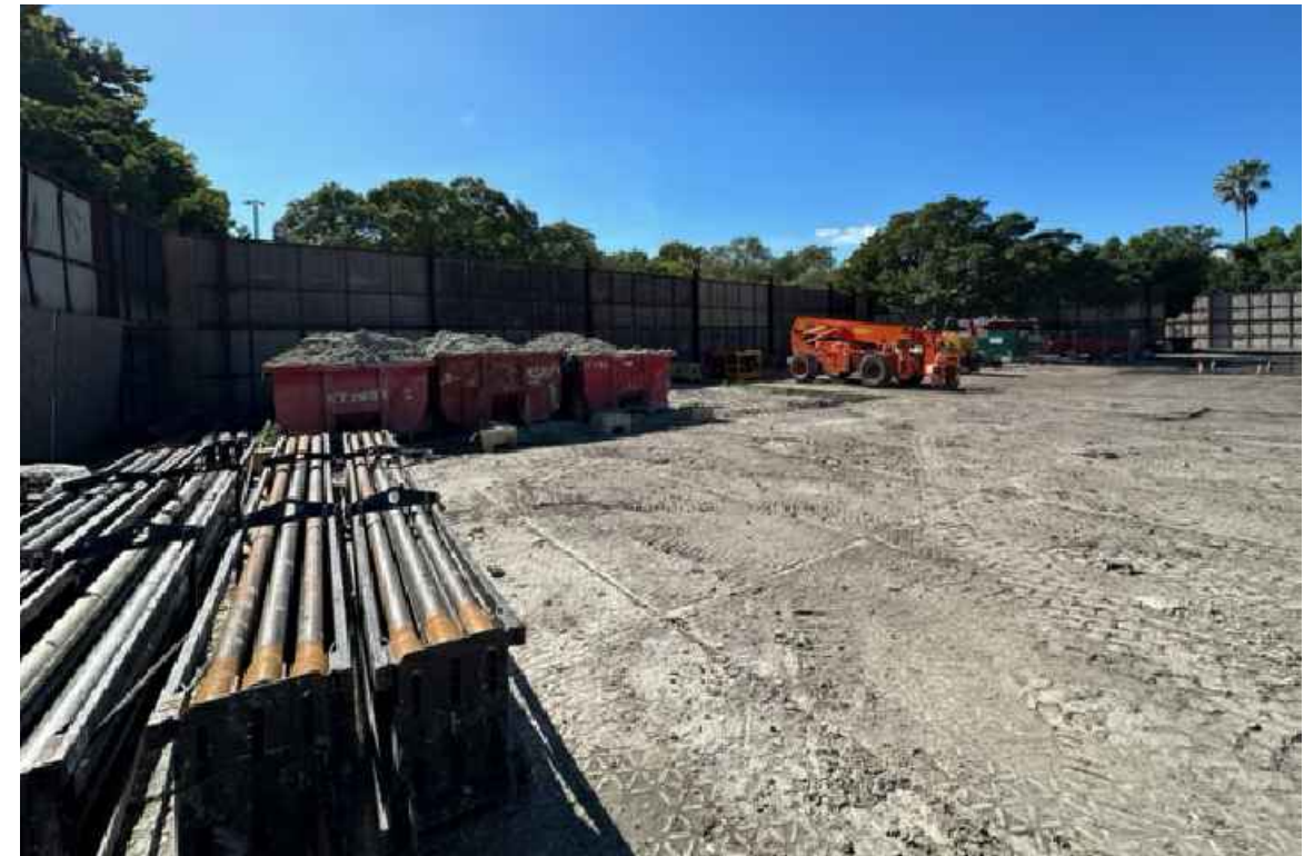
16. INSIDE FPL STAGING AREA FACING MICHIGAN AVENUE
