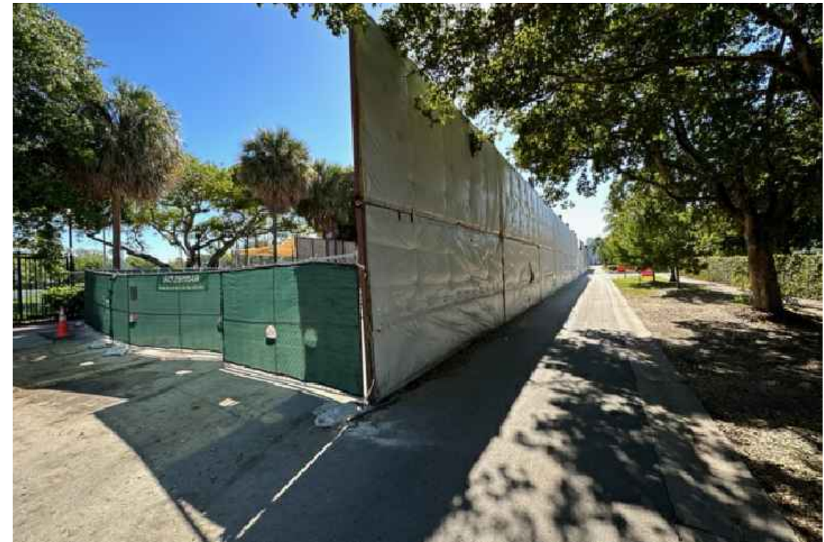
6. FPL WORK ON MICHIGAN AVENUE
