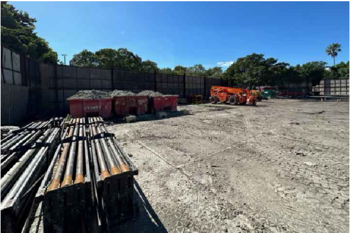
16. INSIDE FPL STAGING AREA FACING MICHIGAN AVENUE
