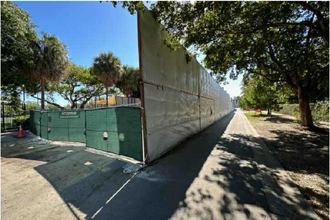
6. FPL WORK ON MICHIGAN AVENUE
