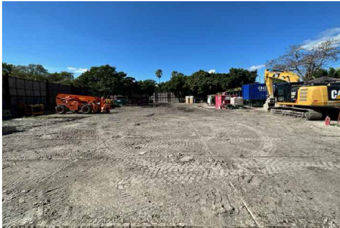
15. INSIDE FPL STAGING AREA FACING MICHIGAN AVENUE
