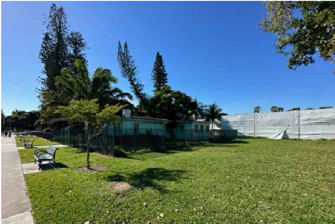
1. LODGING AND FPL STAGING AREA
