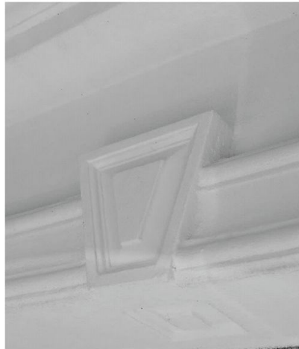
Figure 81. Detail of keystone at garage door, May 2021.
