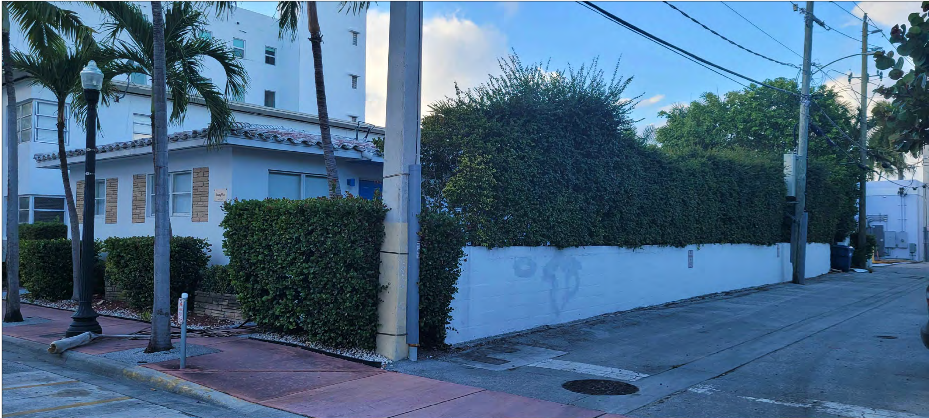
17. ALLEY VIEW FROM SE
