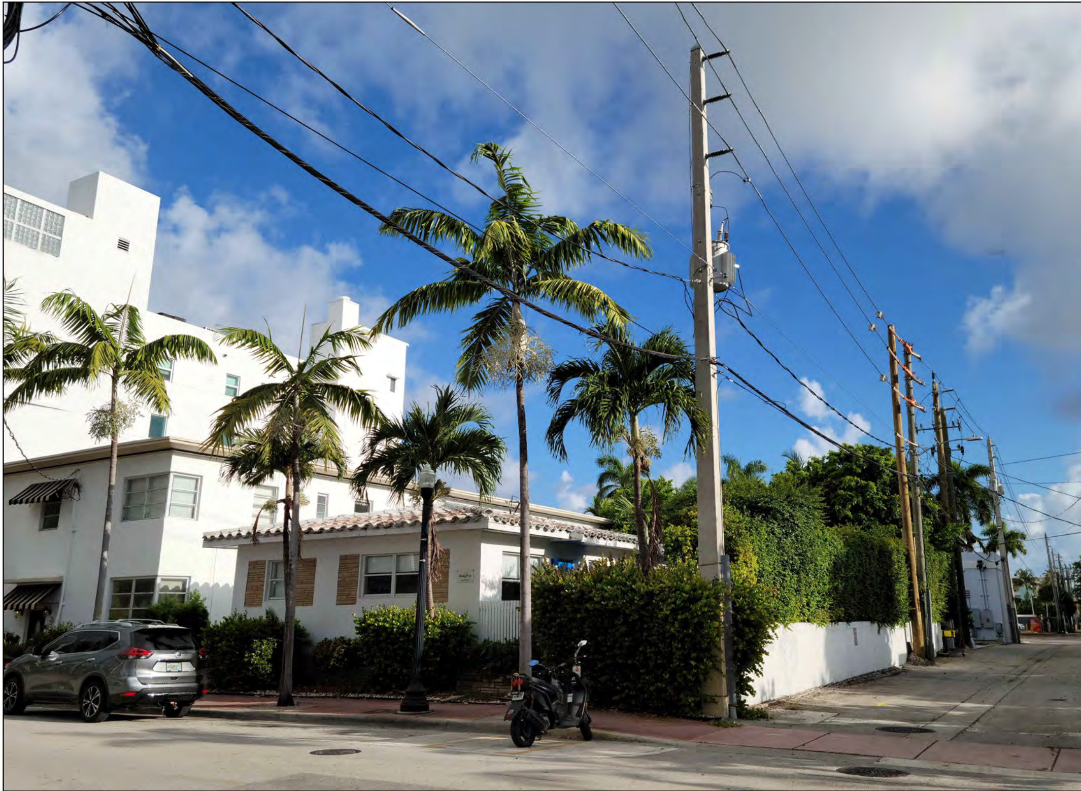
16. STREET FACADE VIEW @ 4TH 5 AND ALLEY
