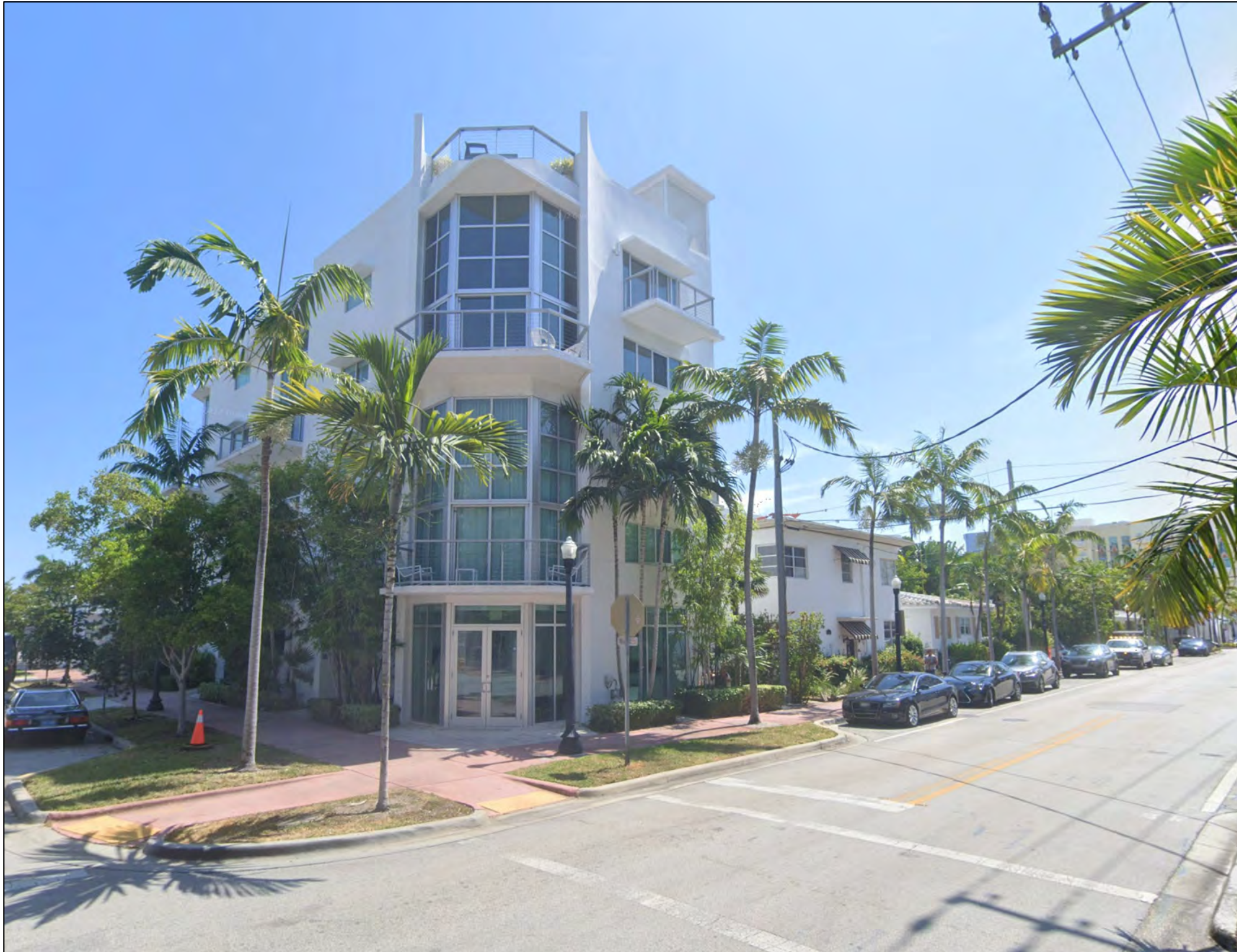
8. STREET VIEW -NORTH SIDE FACING NE
