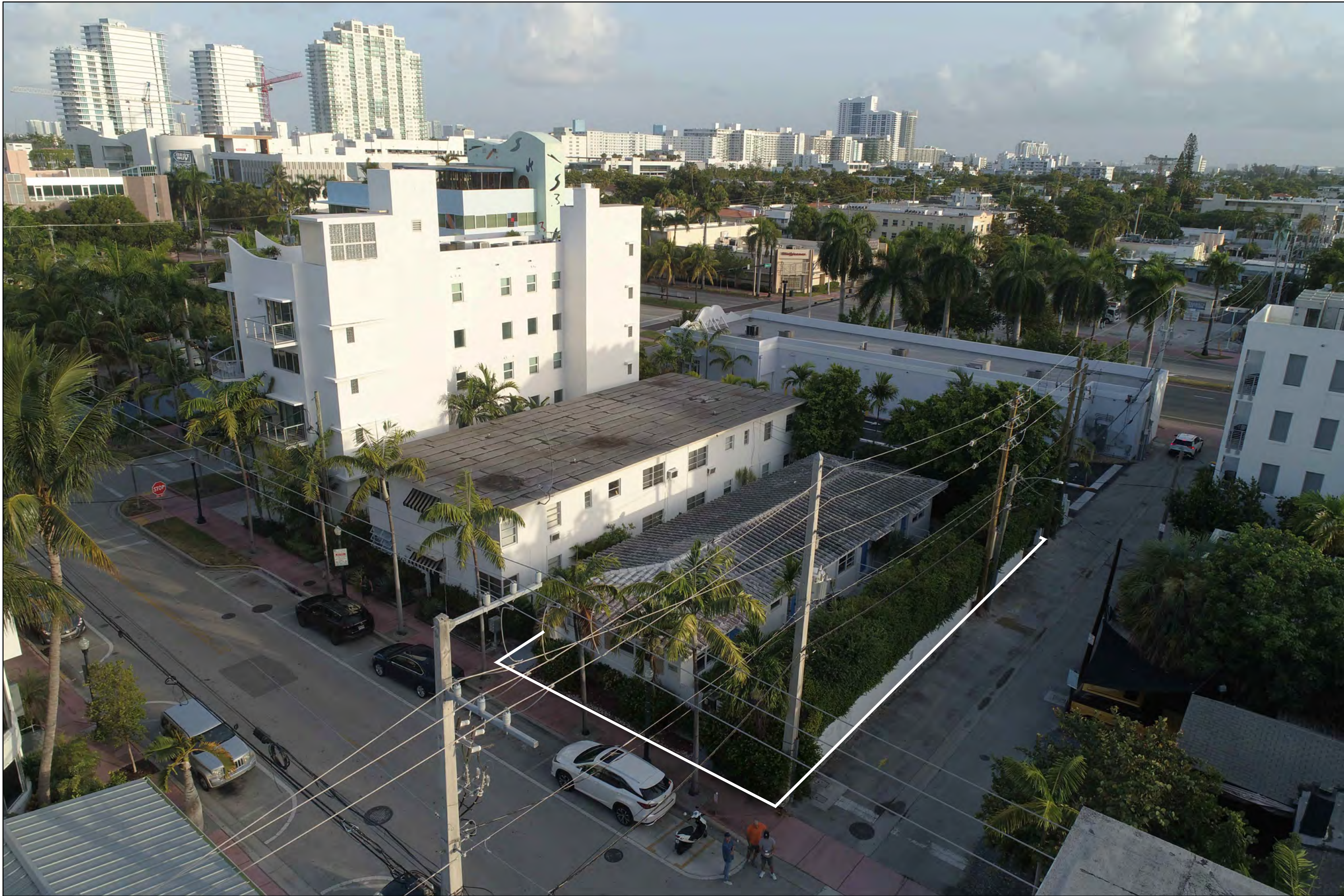
6. AERIAL VIEW OF 829 4TH STREET FACING NW
