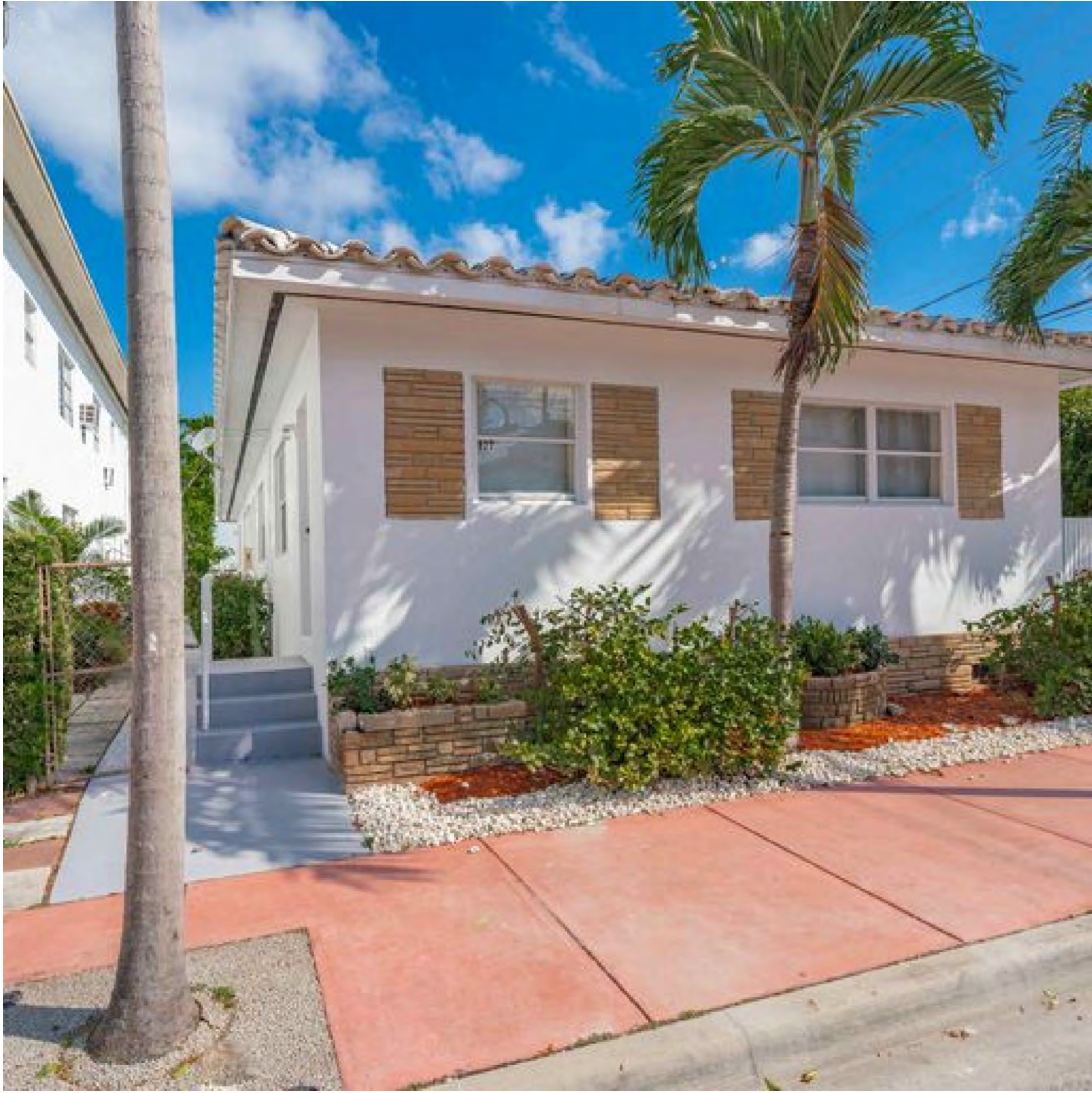
14. STREET FACADE VIEW @ 4TH STREET
