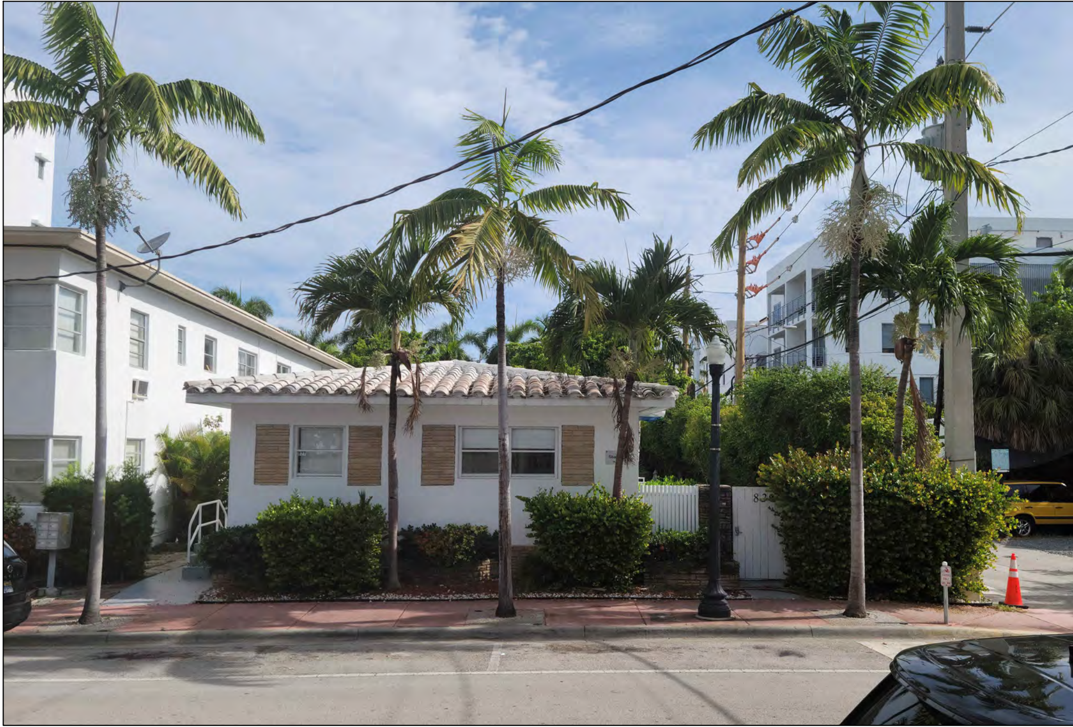
15. STREET FACADE VIEW @ 4TH STREET
