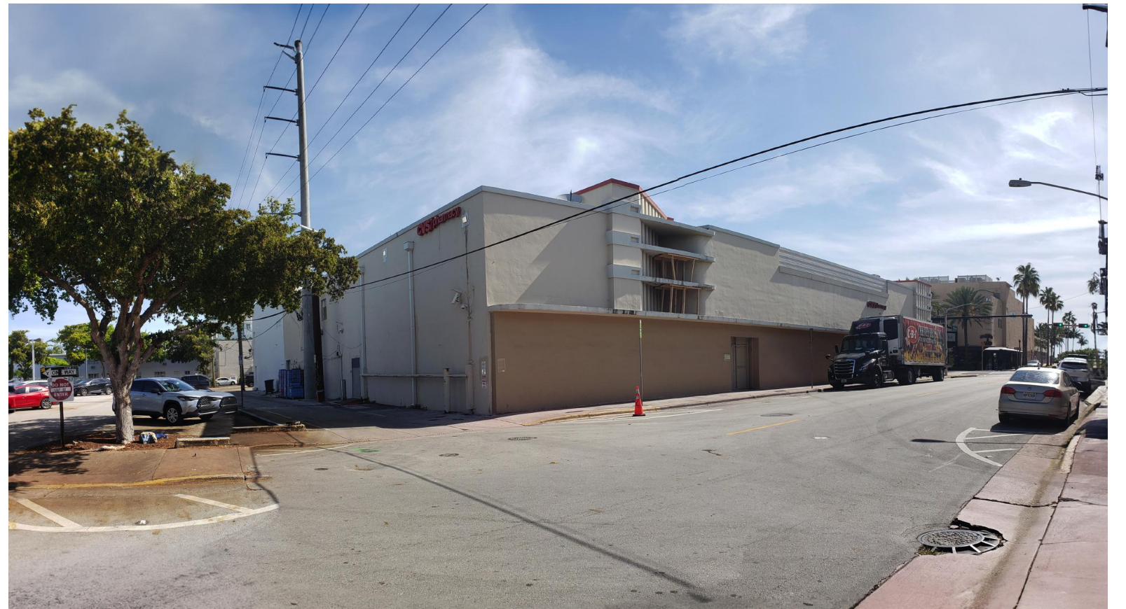
2. CVS Building facing 74 Street
