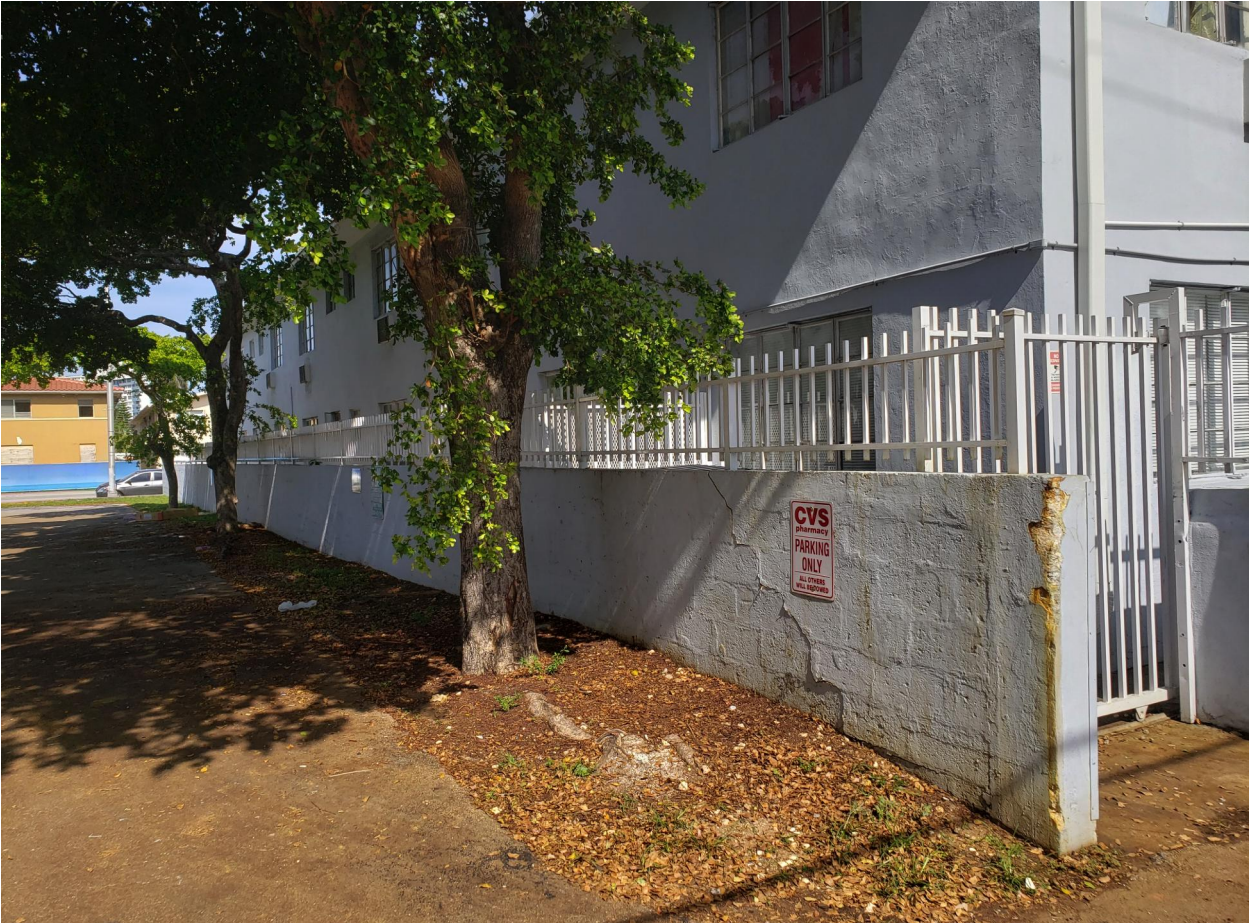
8. Adjacent Neighboring Building
