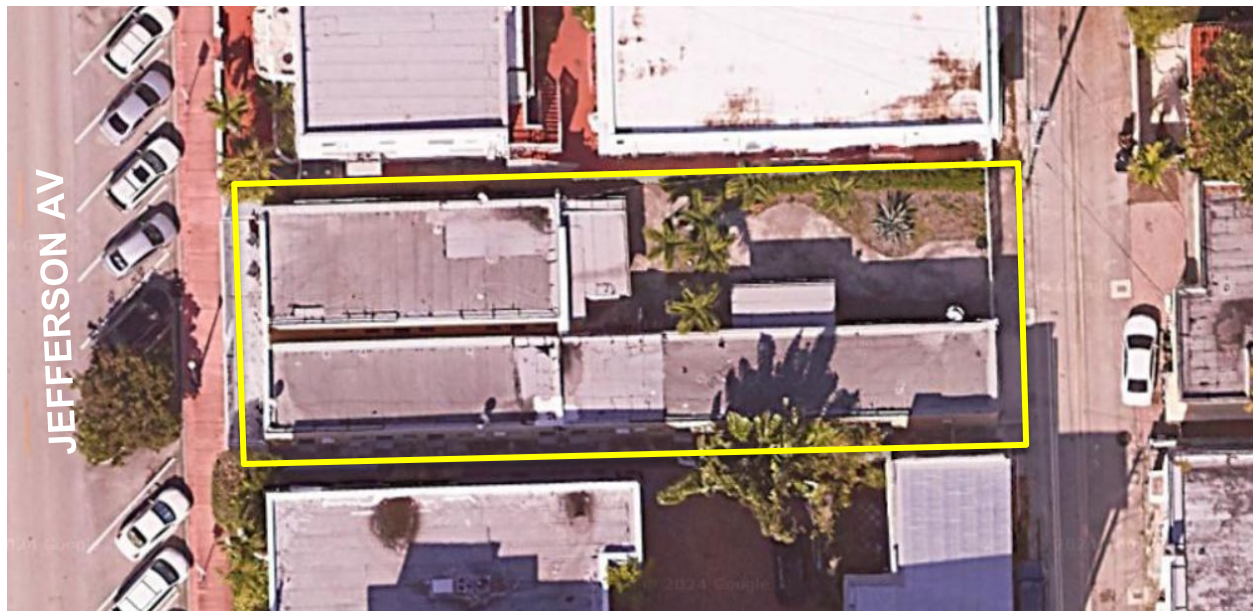
321 Jefferson Avenue aerial, 2024
