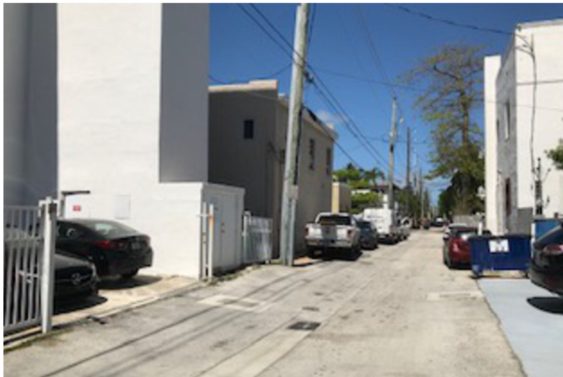
VIEW FROM 4TH STREET LOOKING SOUTH AT MERIDIAN COURT
