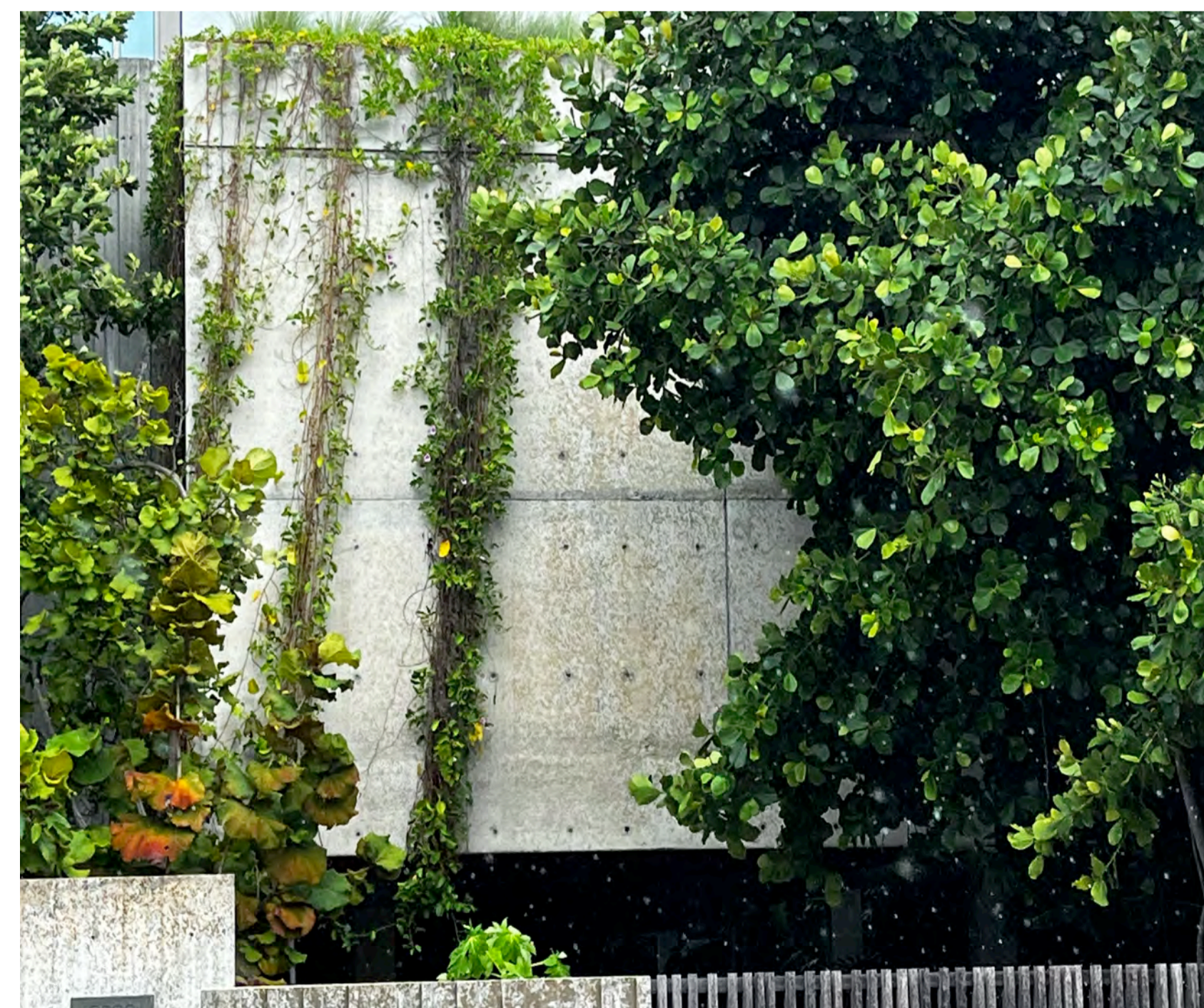
OFF-FORM CONCRETE WALLS
