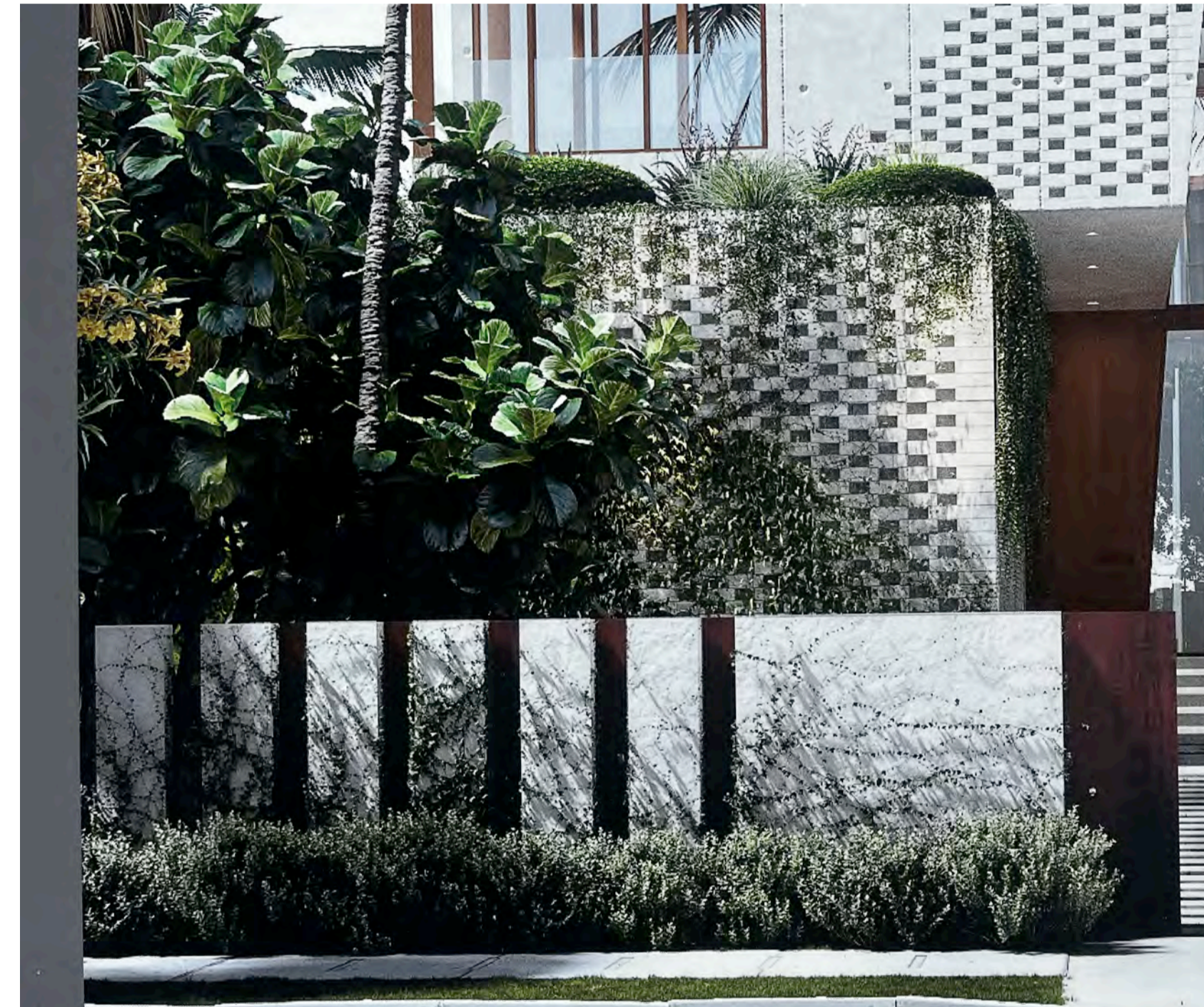
CORTEN STEEL & CONCRETE FENCE
