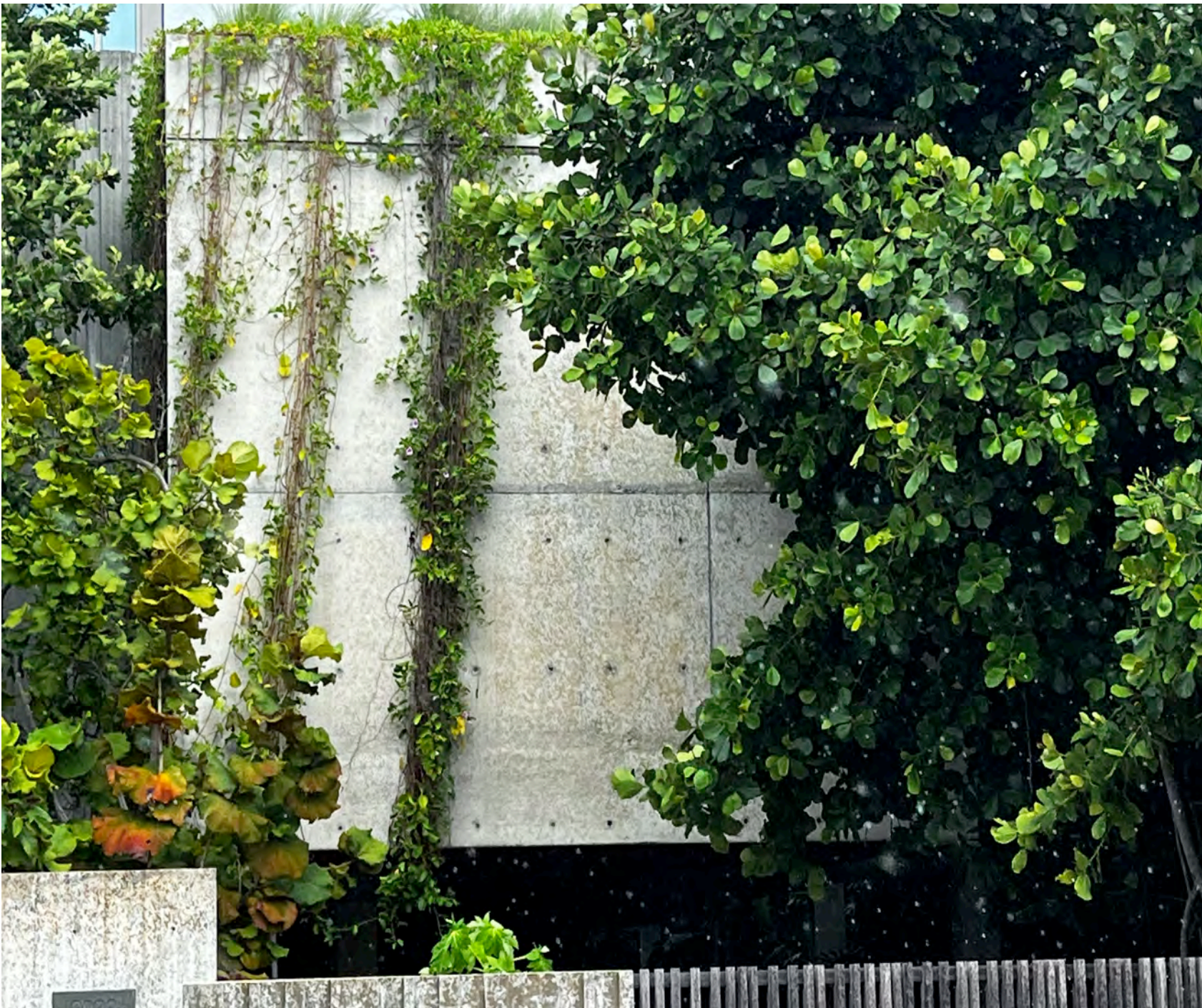
OFF-FORM CONCRETE WALLS
