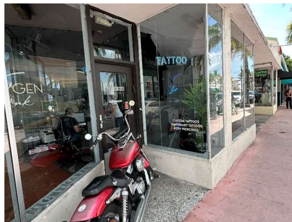
Figure 84. Detail of entrance to 1523 Washington Avenue, August 2023.
