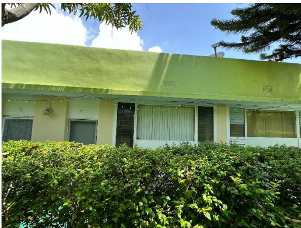
Figure 101. View of Unit 10, looking north, August 2023.
