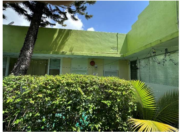
Figure 100. View of Units 8 and 9, looking northeast, August 2023.
