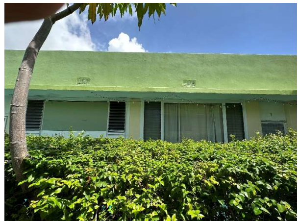
Figure 102. View of Unit 11, looking north, August 2023.
