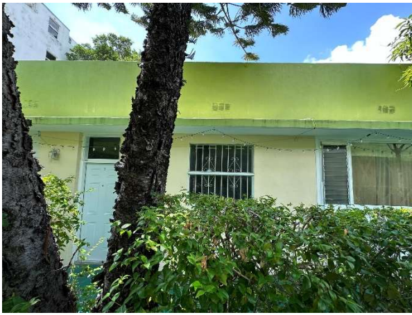
Figure 97. View of Unit 5, looking south, August 2023.
