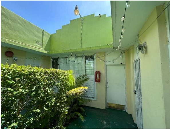
Figure 99. View of Unit 7, looking east, August 2023.
