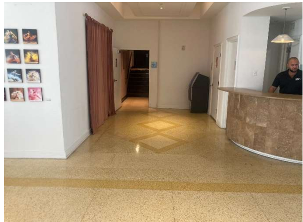
Figure 31. Detail of terrazzo flooring, September 2023.
