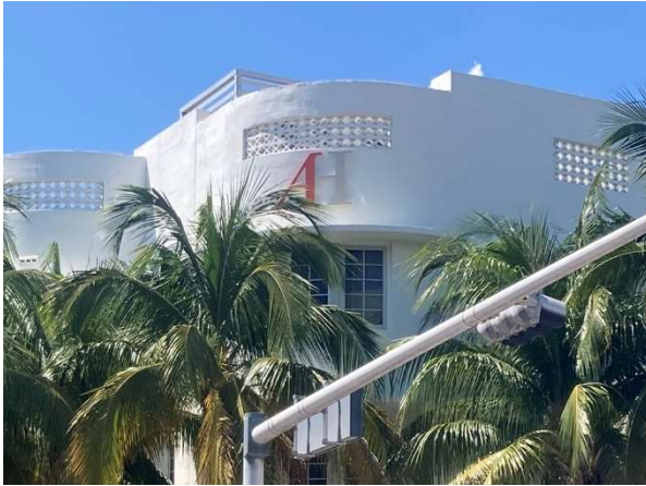
Figure 28. Detail of breeze block, September 2023.
