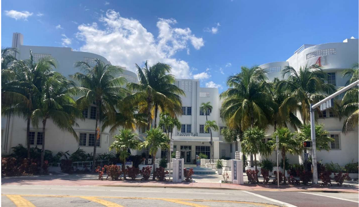
Figure 25. View of 1500 Collins Avenue, looking west, September 2023.
