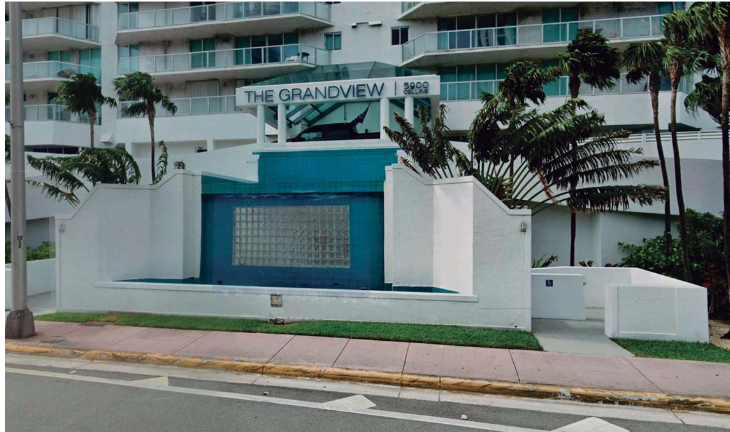
1 A-0.5 EXISTING FOUNTAIN CONDITION
