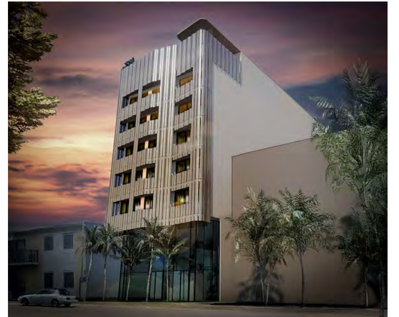
NW VIEW (FRONT) - NIGHTTIME
