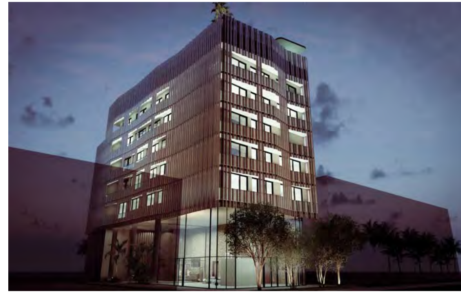
NW VIEW (FRONT) - NIGHTTIME
