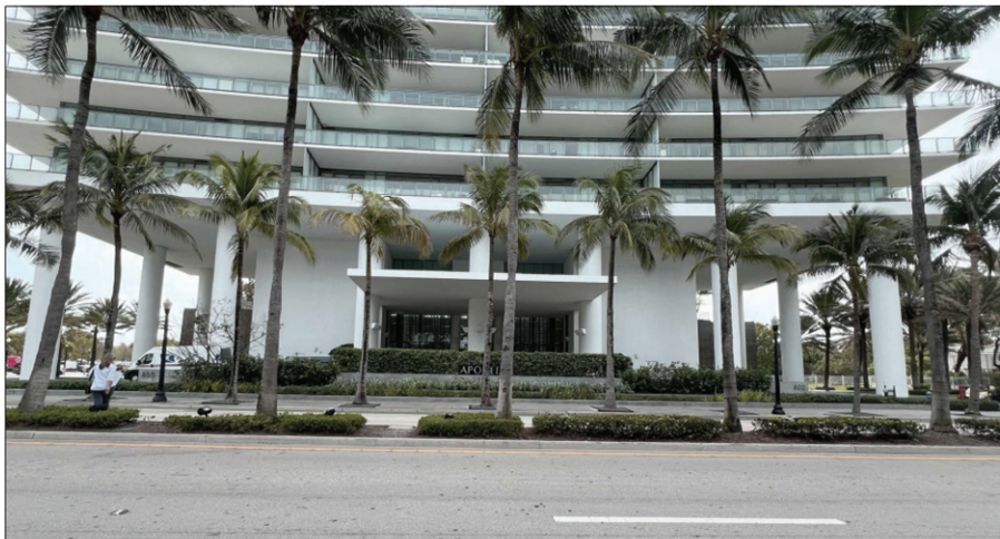
SITE VISIT 1/25/2024 3) VIEW OF NORTH ELEVATION
