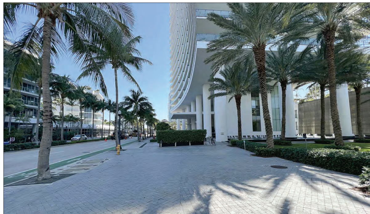
SITE VISIT 3/01/2024 4) NE PROPERTY CORNER VIEW EAST
