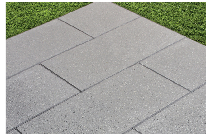
DRIVEWAY HARDSCAPE MATERIAL
