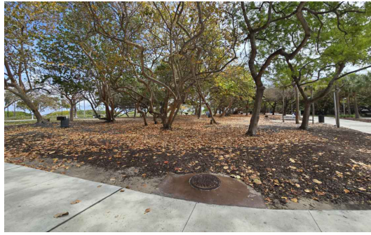
7. BBQ GRILL AND SANITARY MANHOLE - SE VIEW
