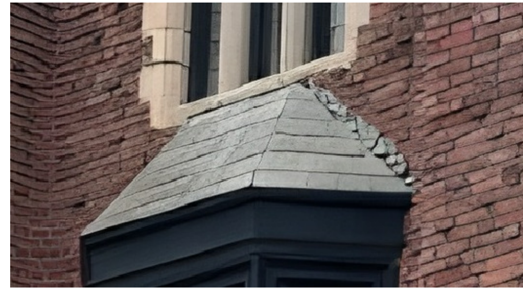
EXISTING SLAT ROOF
