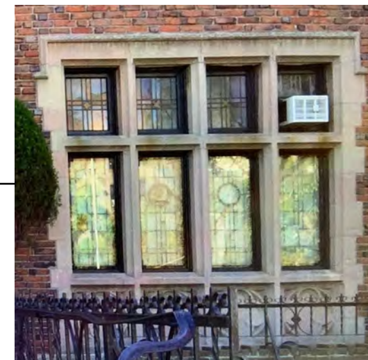
PRECAST STONE MOULDING AROUND WINDOW
