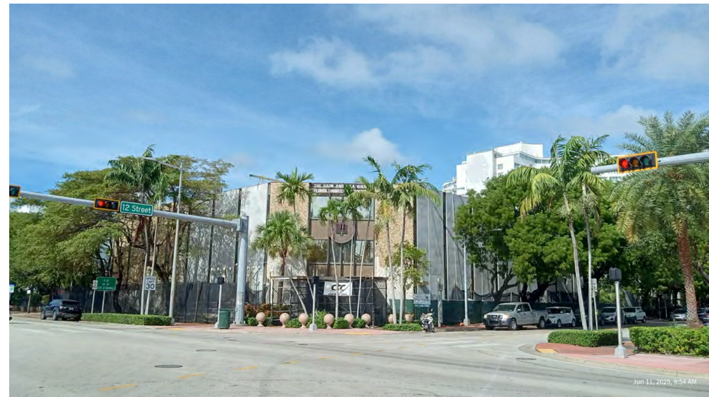
2) CORNER FACADE VIEW FROM ALTON ROAD
