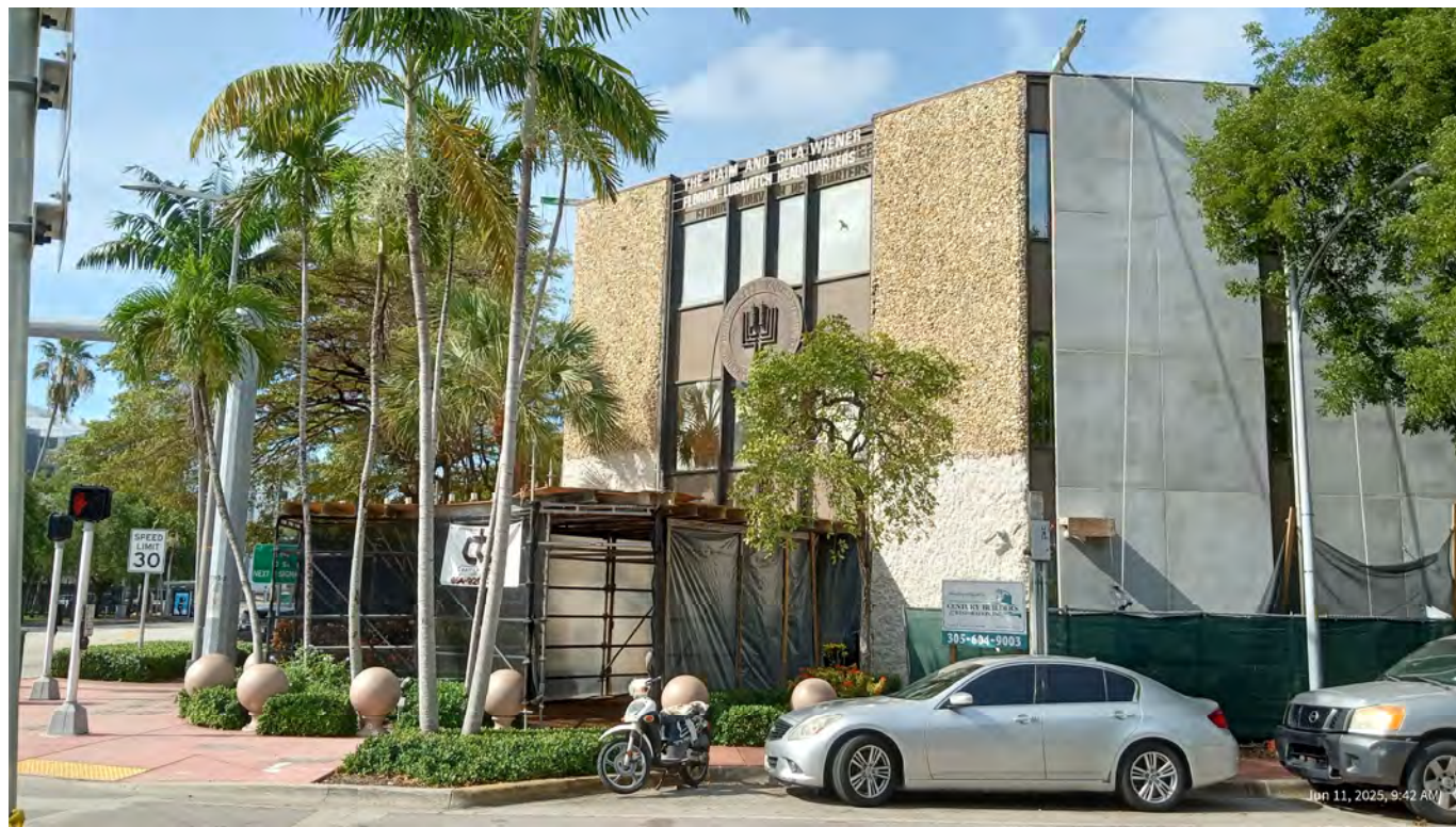
1) CORNER EXISTING FACADE
