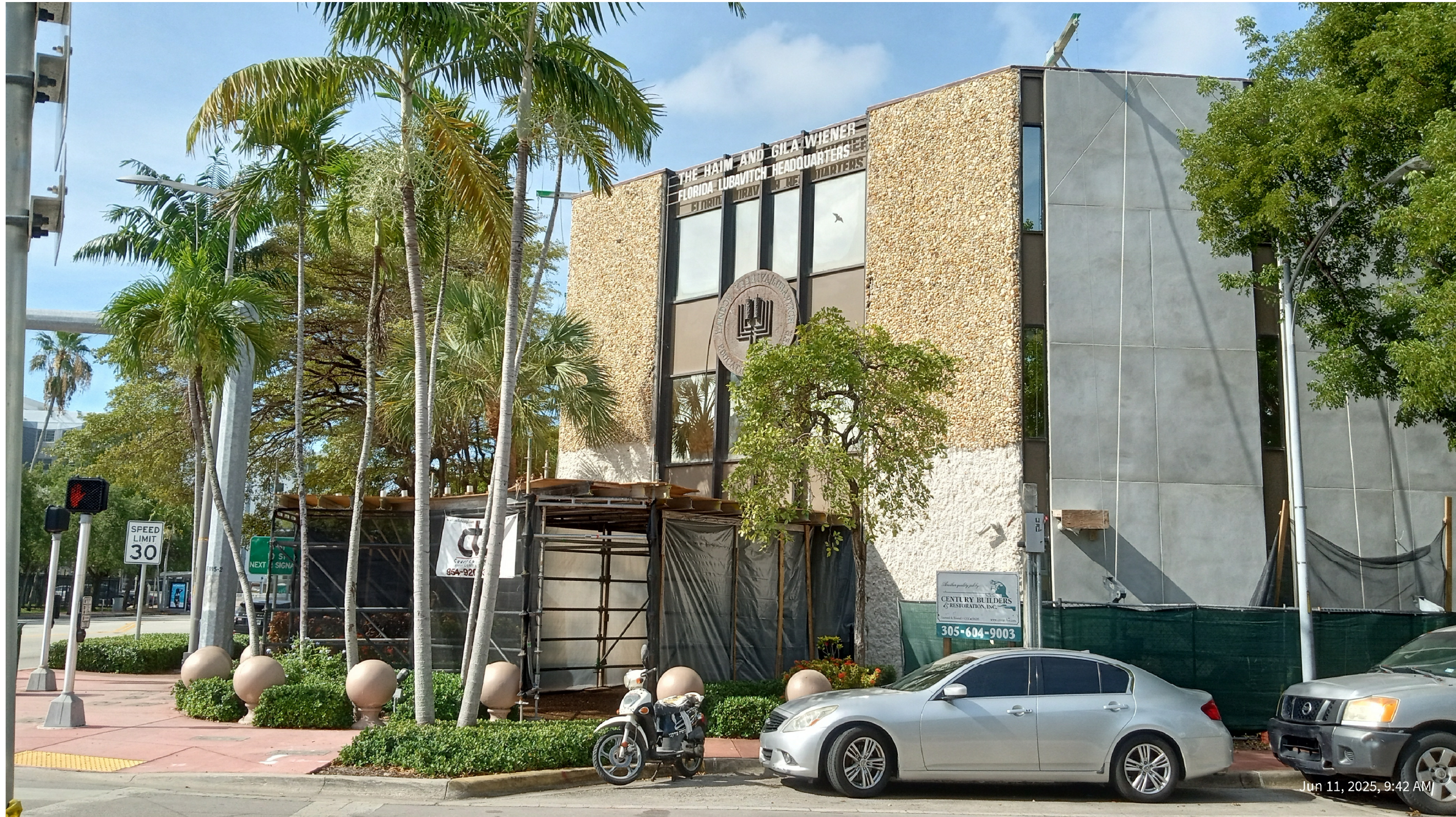
CORNER EXISTING FACADE
