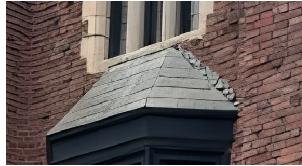
EXISTING SLAT ROOF
