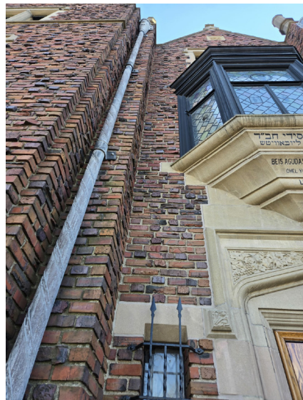
PRECAST STONE MOULDING
