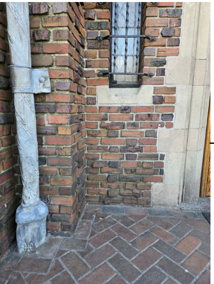
PRECAST STONE MOULDING AND BRICK
