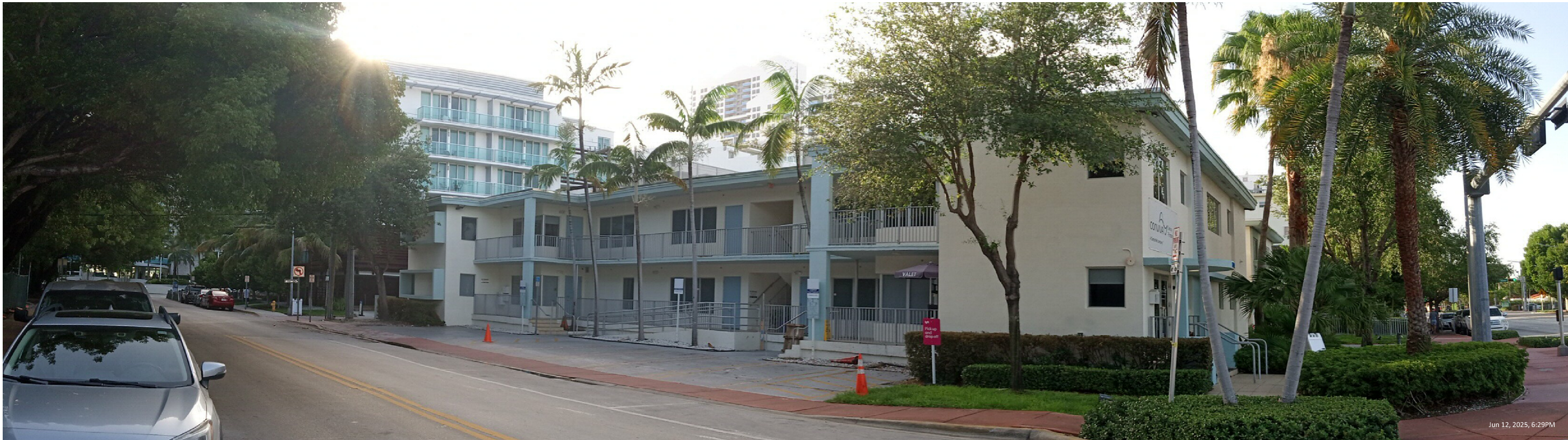
CONTEXTURAL PANORAMIC ALONG 12 TH STREET - LOOKING NORTH
