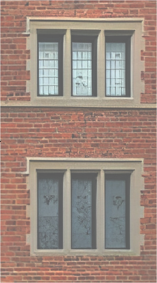
PRECAST STONE MOULDING AROUND WINDOWS
