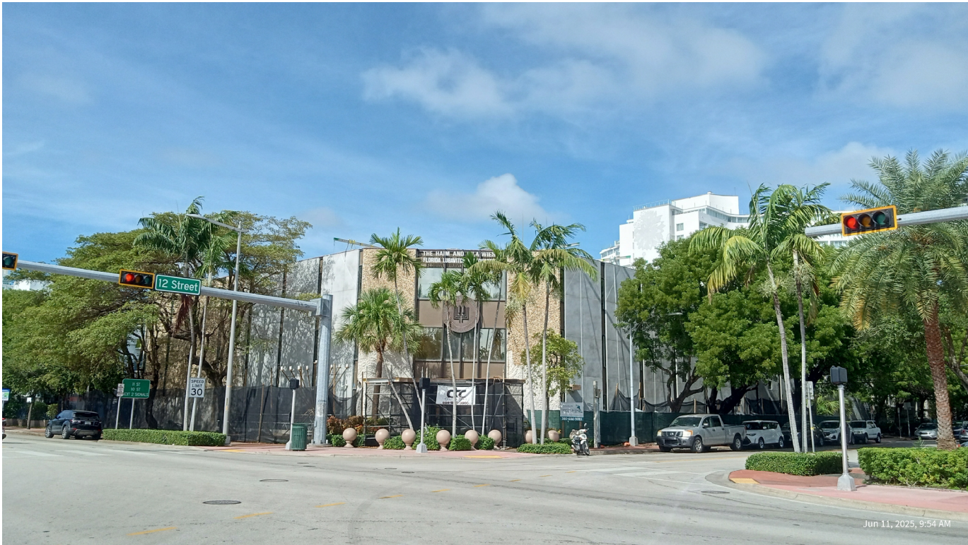
2) CORNER FACADE VIEW FROM ALTON ROAD
