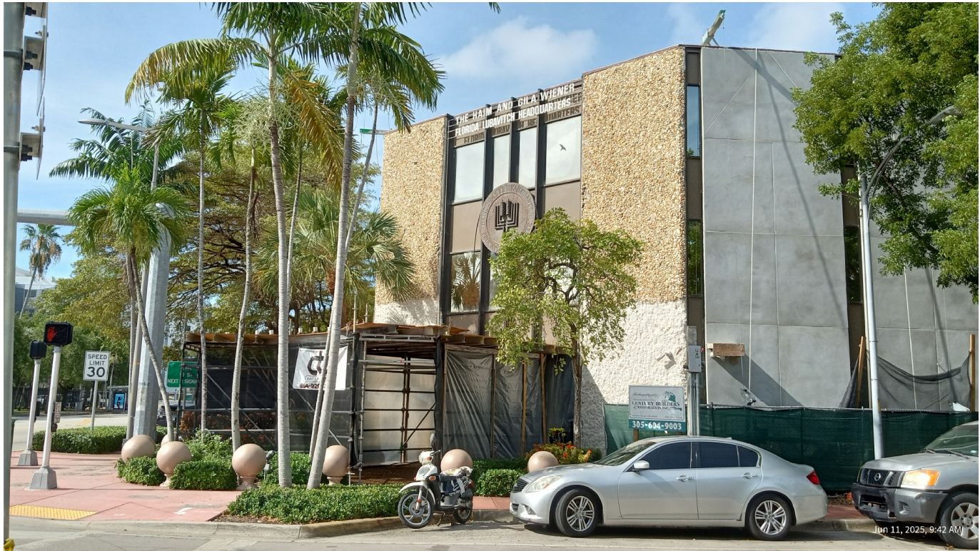
1) CORNER EXISTING FACADE
