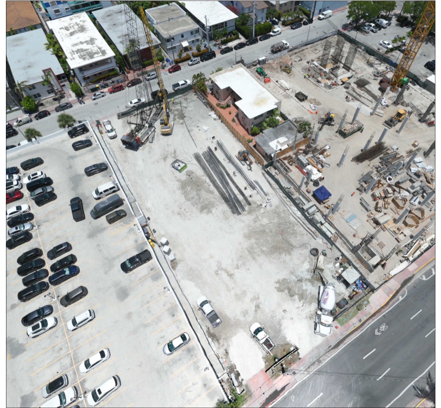
VIEWS TOWARDS WEST
