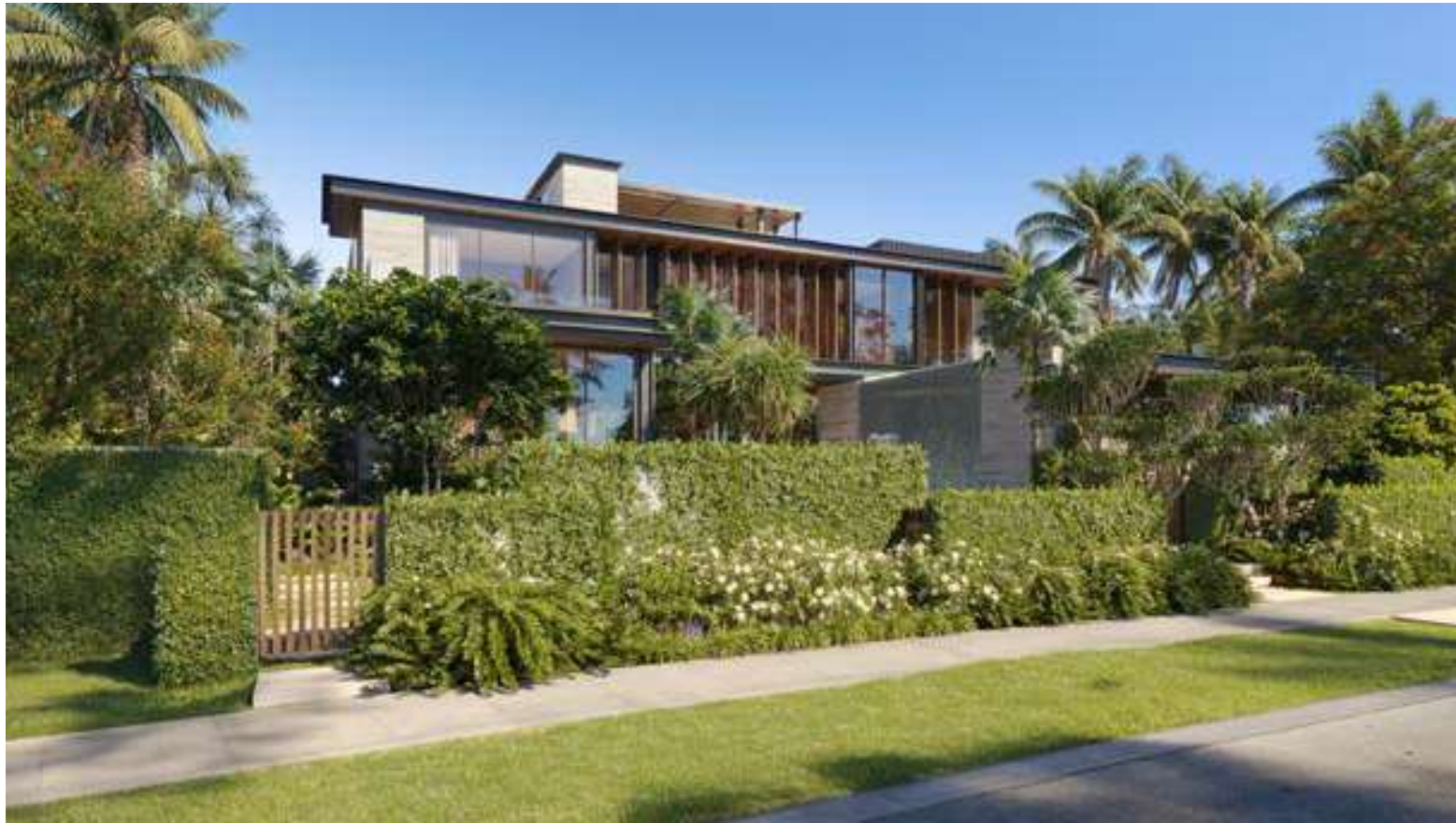
FRONT OVERALL _ FROM DIDILO DR. [LOOKING NORTHWEST]
