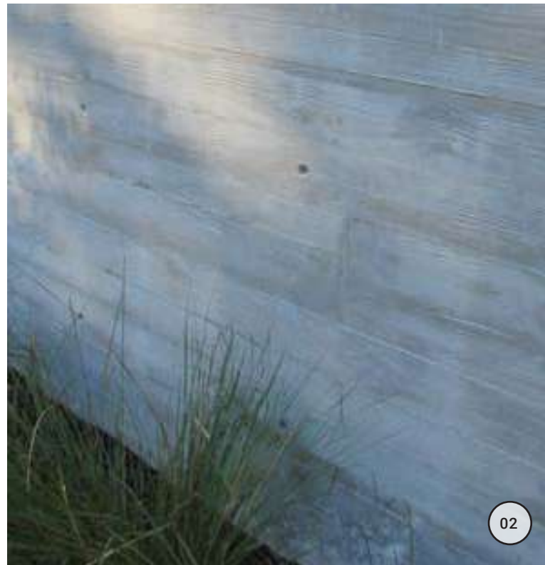
BOARD FORMED CONCRETE
