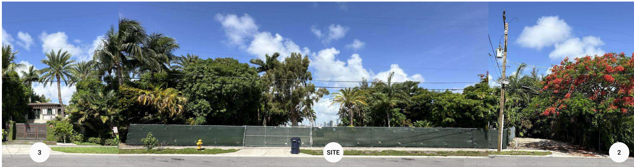
EXISTING CONDITION - FRONT OF RESIDENCE W/ SURROUNDING CONTEXT
