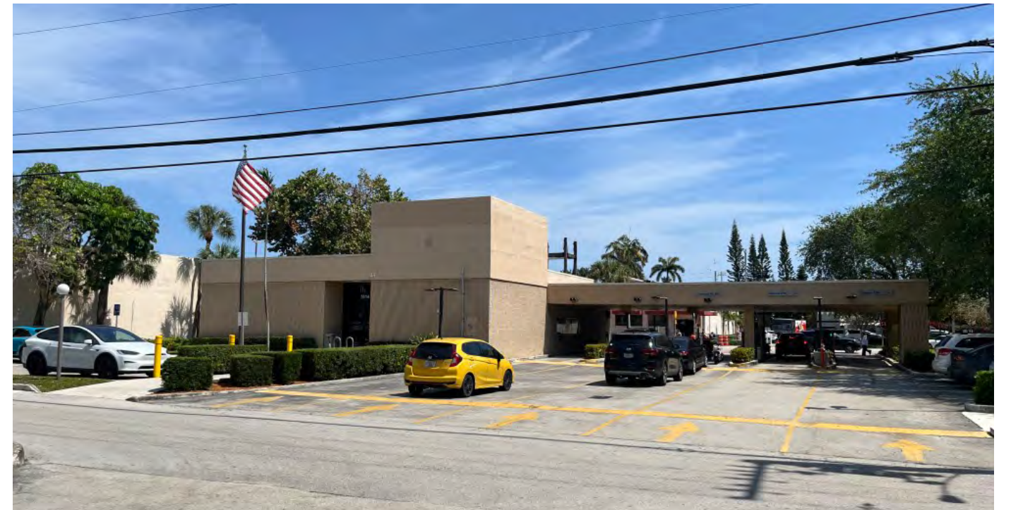
02 - VIEW OF EXISTING STRUCTURE FROM ALTON COURT - WEST
