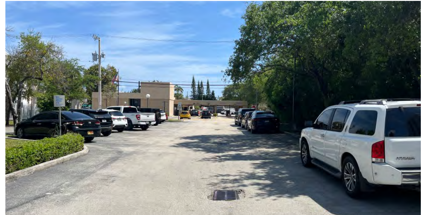
02 - VIEW OF EXISTING STRUCTURE FROM WEST AVE
