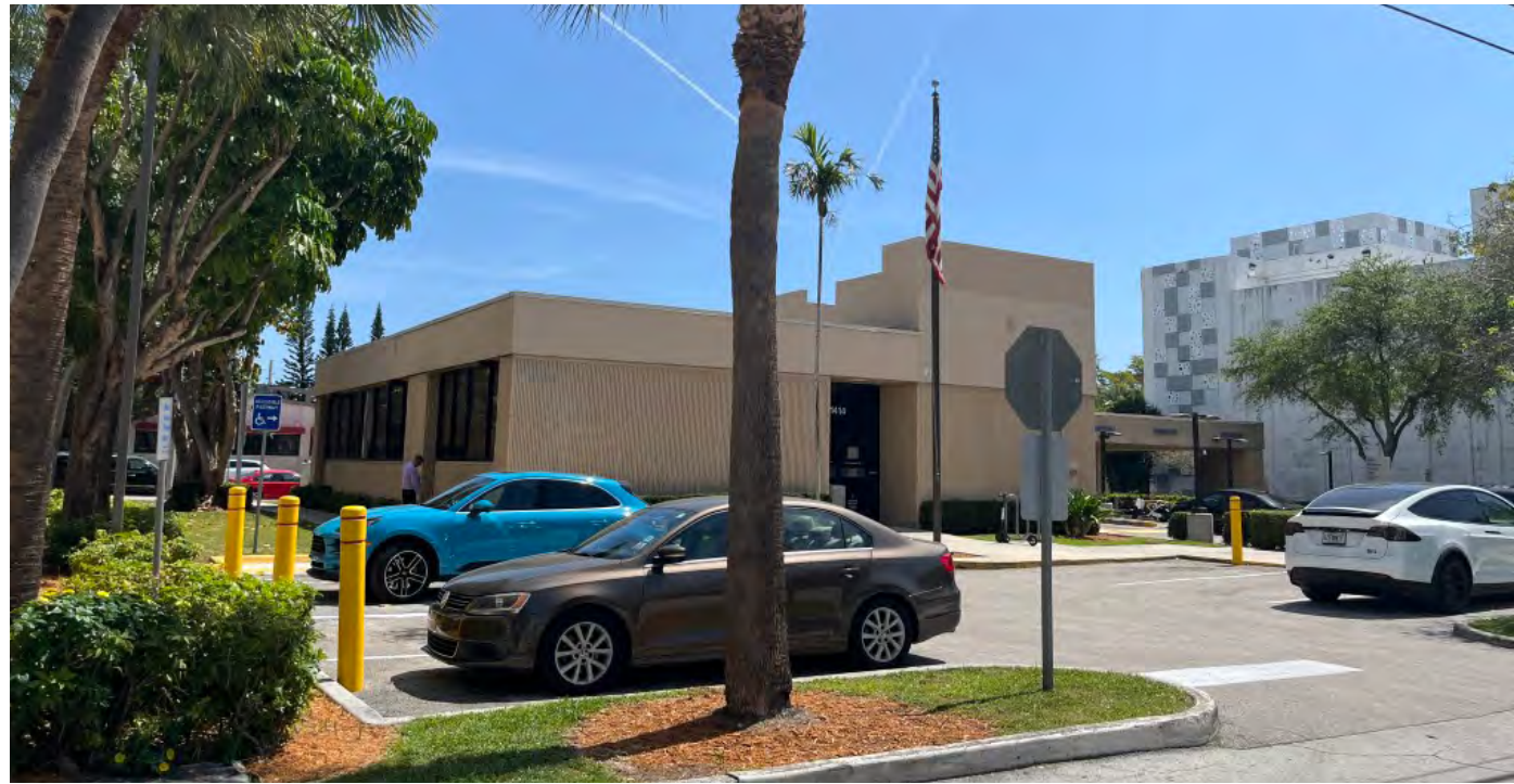
01 - VIEW OF EXISTING STRUCTURE FROM ALTON COURT - NORTH
