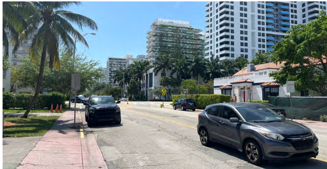
03 - VIEW OF WEST AVE - SOUTH
