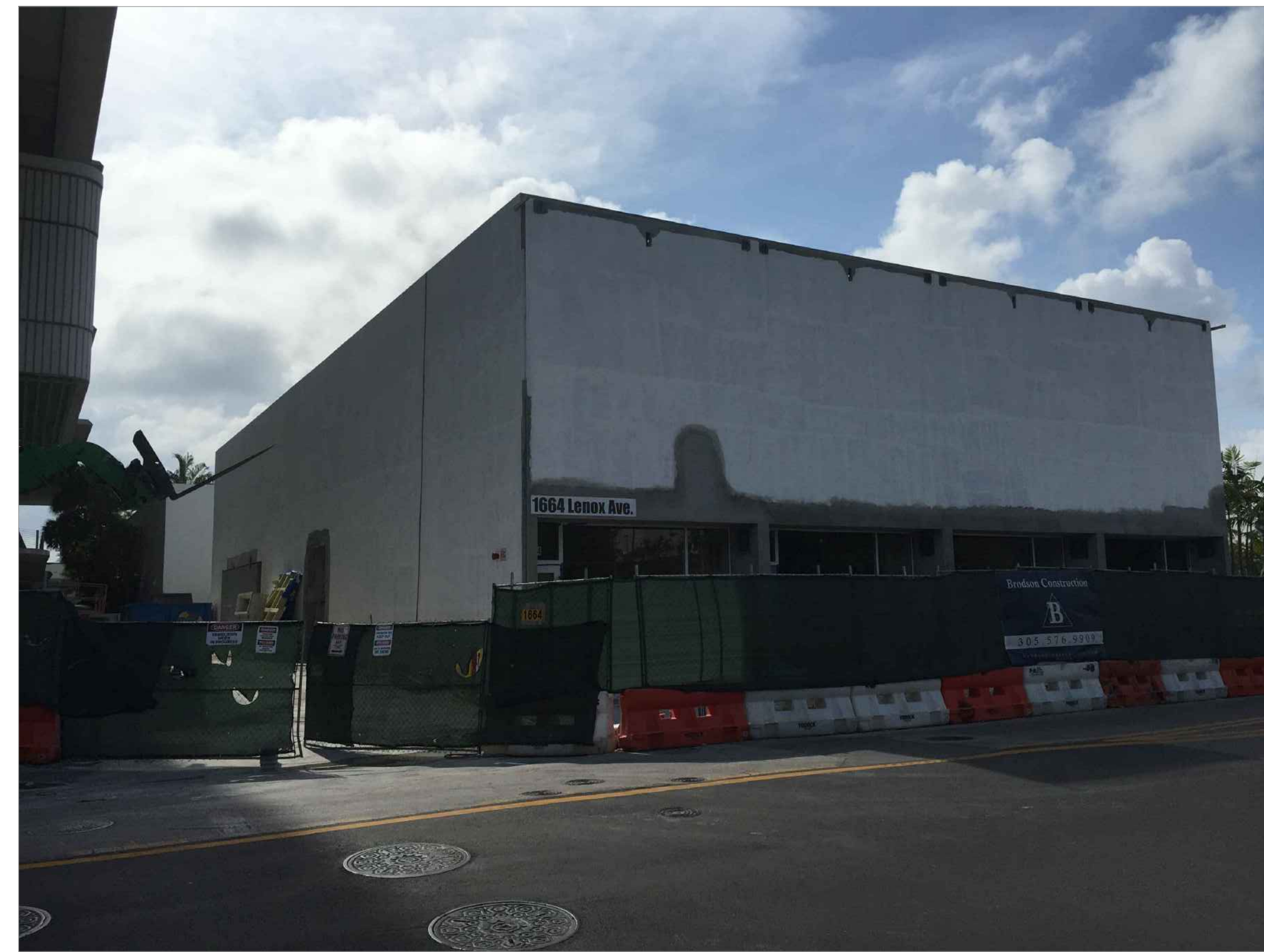
SOUTH EAST CORNER OF SUBJECT PROPERTY
