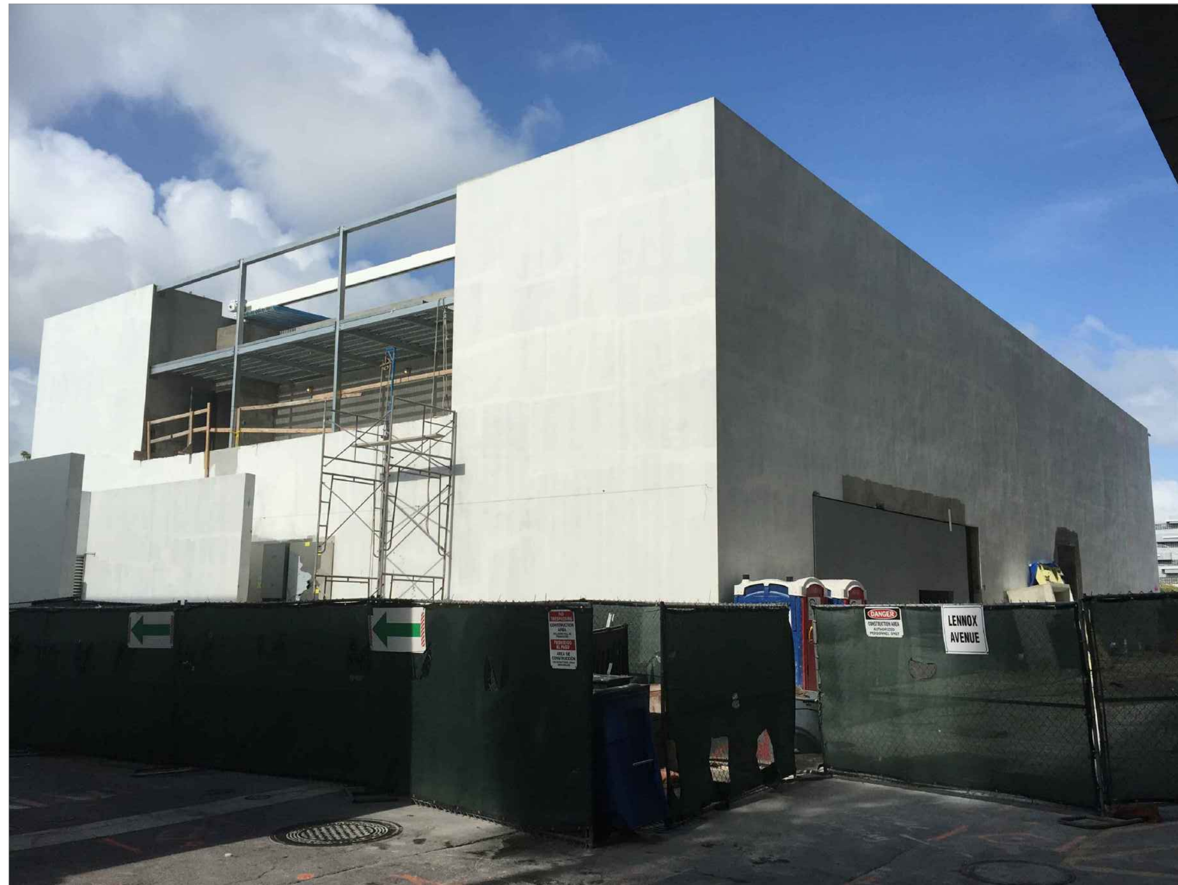
SOUTH WEST CORNER OF SUBJECT PROPERTY
