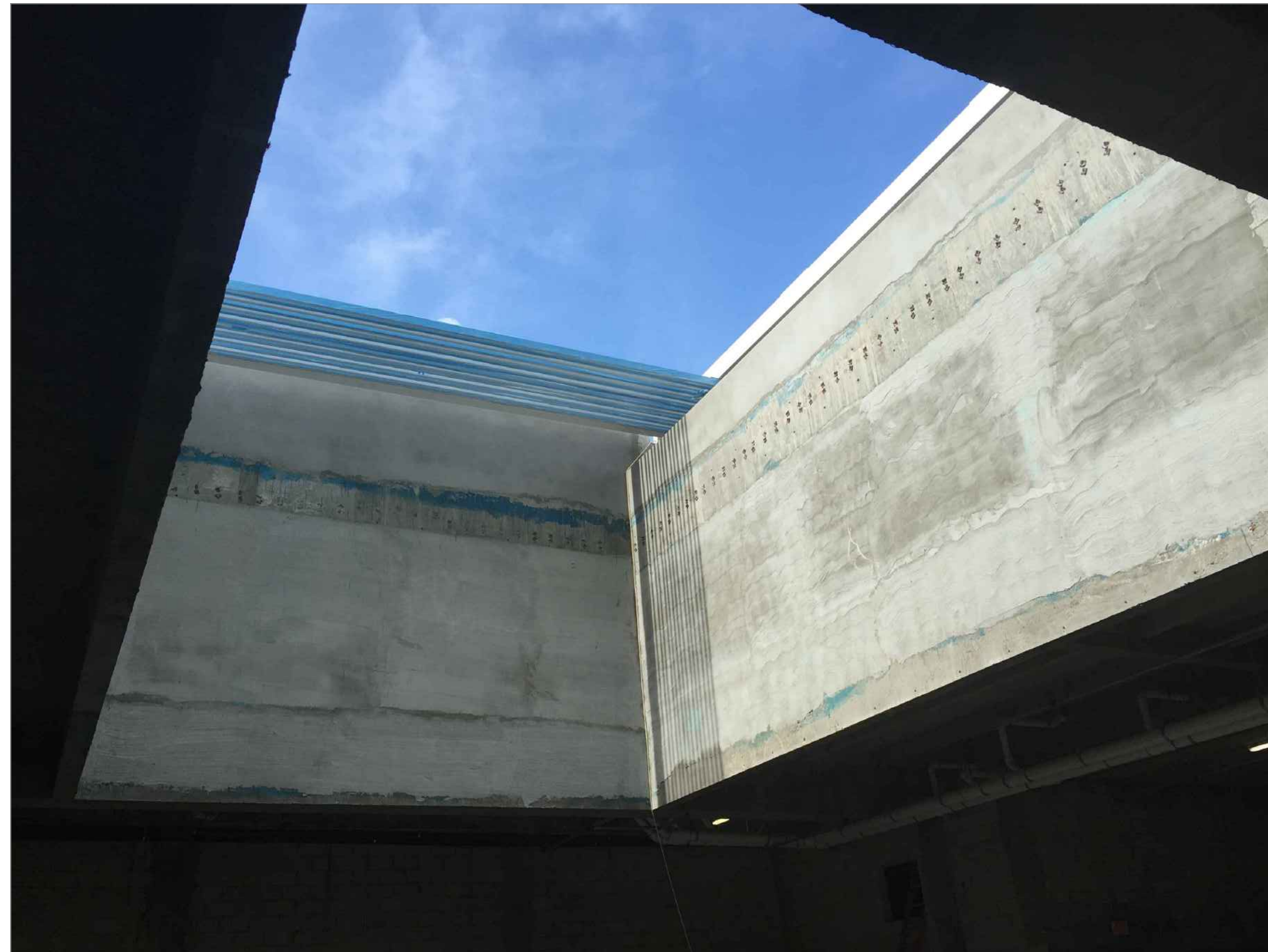
INTERIOR: NORTH EAST VIEW OF ROOF OPENING
