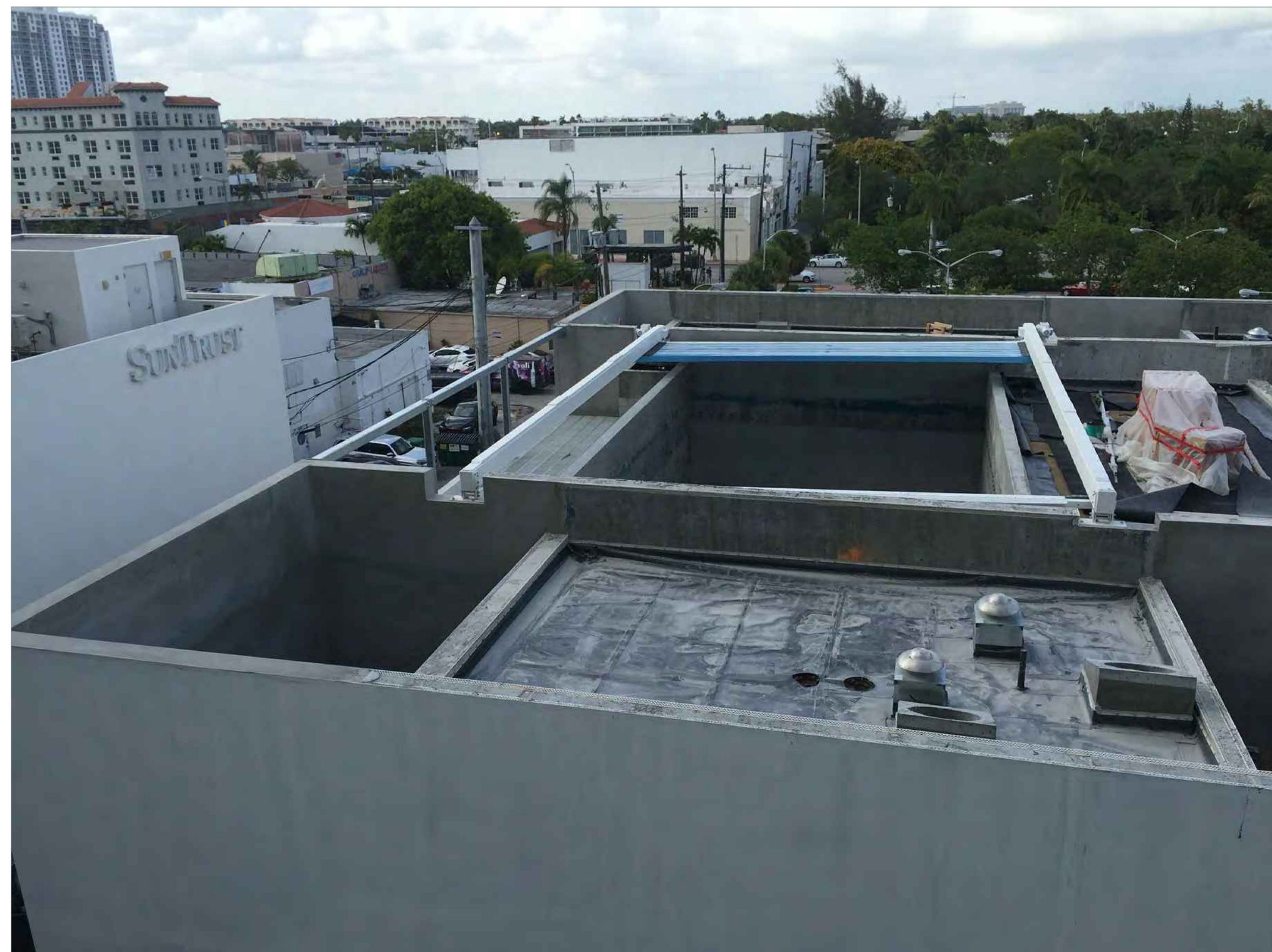
ROOF: WEST END VIEW
