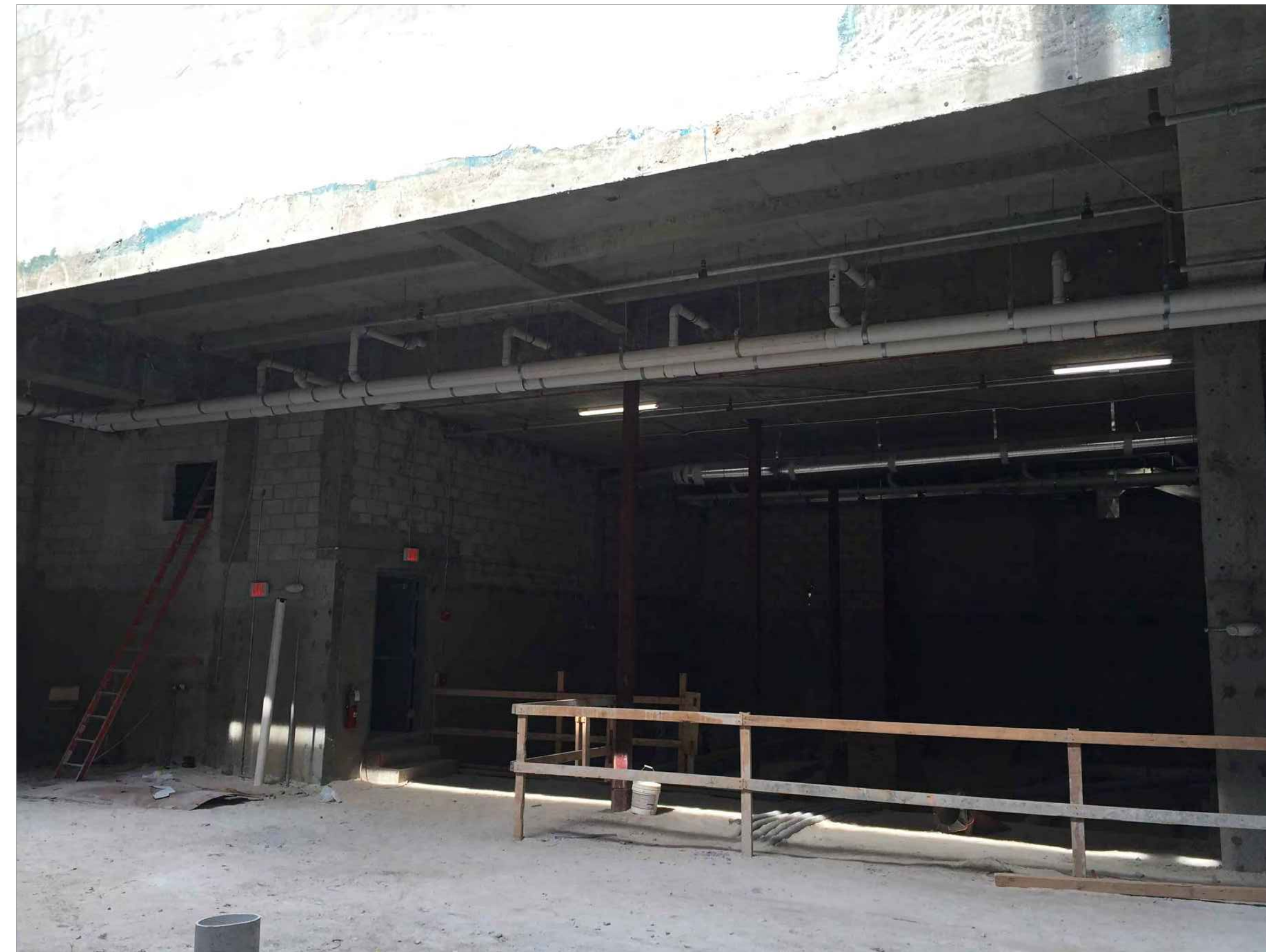
INTERIOR: EAST VIEW
