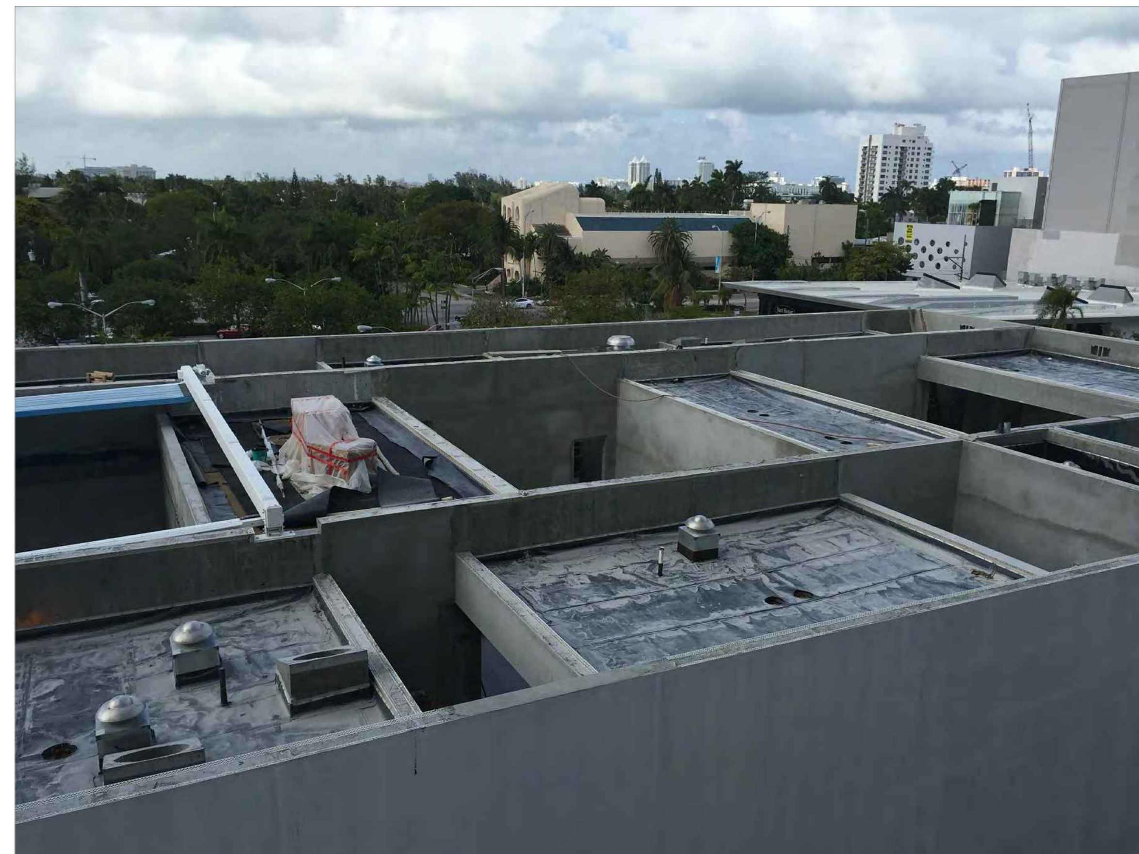
ROOF: CENTER AND EAST VIEW
