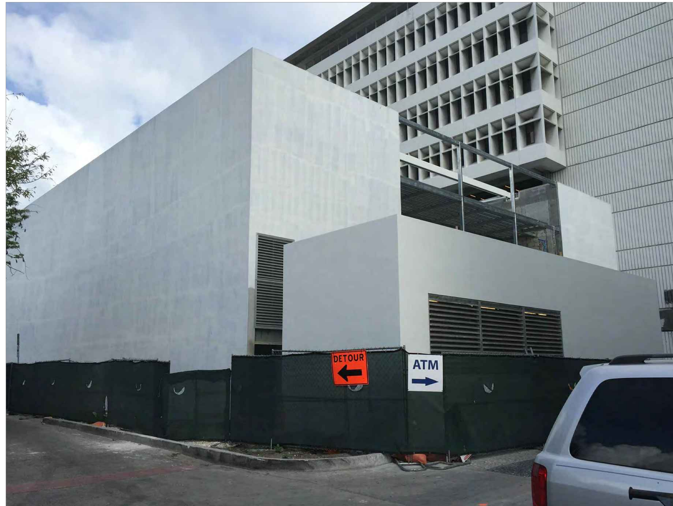
NORTH WEST CORNER OF SUBJECT PROPERTY
