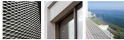
MS-01 ALUMINUM MECHANICAL SCREEN GL-01 IMPACT GLAZING - CLEAR W/ BRONZE FRAME GLR IMPACT GLASS HANDRAIL - CLEAR
